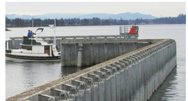
Partially penetrating wave barrier
