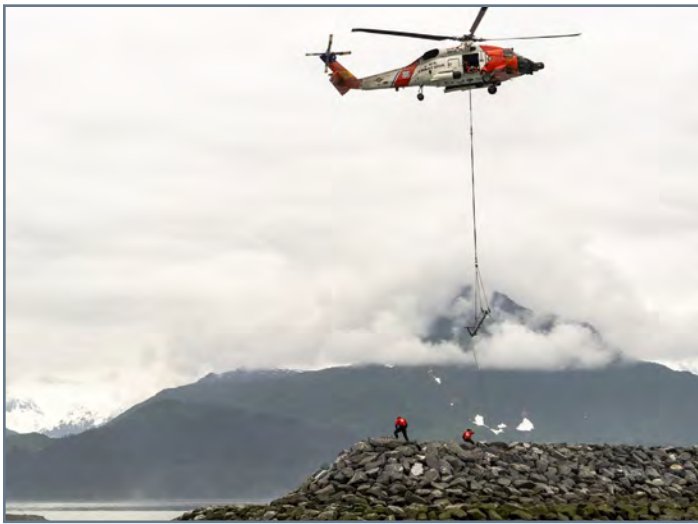
Coast Guard helicopter lowering a Navigation Aid to crew for installing at harbor entrance. Photo courtesy of J. Talbott.
