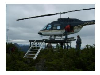
See photos for examples of the portable/removable helipads. They can be constructed on site, or flown in, and easily adapt to undulating or sloping land.
