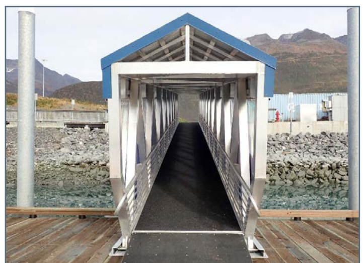
Gangway with metal roof and nonslip transition to the float
