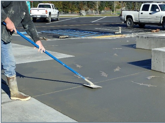
Finishing concrete with fish inlays east of Warehouse Building
