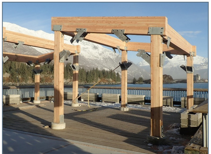
Partially erected timber structure for east Picnic Canopy
