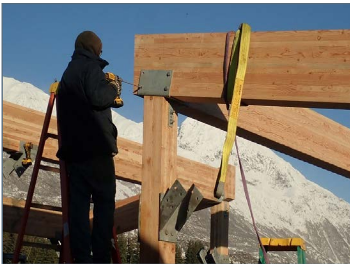
Connecting timbers with brackets for the east Picnic Canopy
