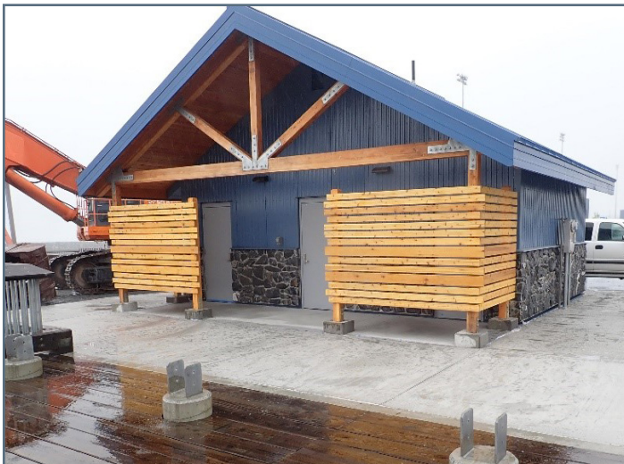
Wood wind screen and sidewalks installed at East Restroom
