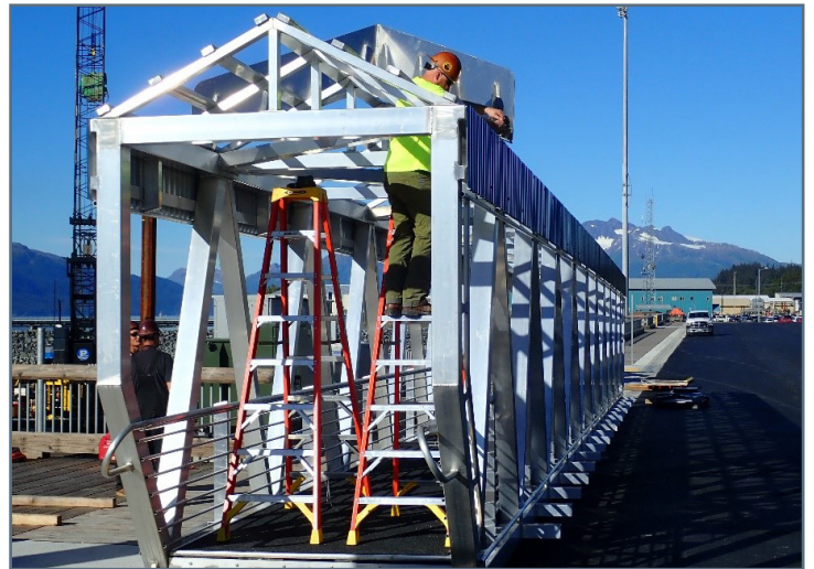
Installing canopy, then side panels, on Gangway #1
