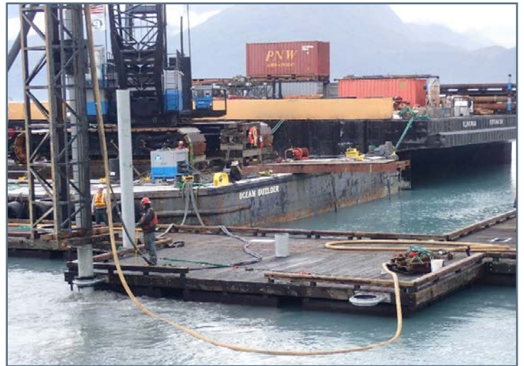
Drilling into bedrock to install piling for Gangway #2
