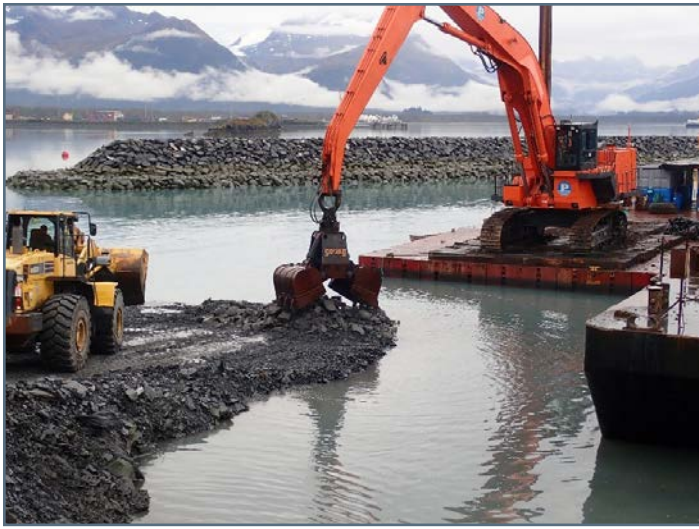
Loading rock on barge for placing on sides of Drive-down basin
