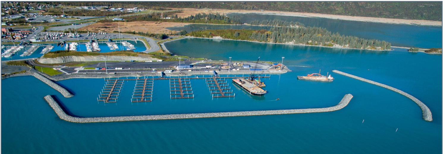
Aerial view after installing 80% of the floats in the Mooring Basin. Piling and floats delivered on the large barge (right of center) were unloaded with crane and installed with piling driven by equipment on smaller barge (tied behind). Dredge equipment and bottom dump barge are located at east (right) end of the Uplands and the Drive-Down Float Basin. (J Talbott, 10/01/18)
