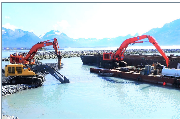
Breaking and excavating rock for dredging and disposing
