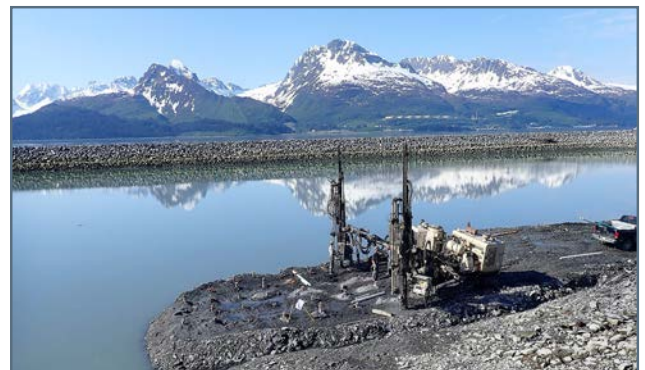
Drilling holes for blasting rock at the West part of mooring basin
