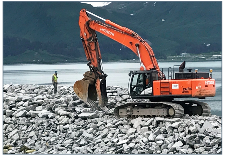
Placing armor rock on Stub Breakwater
