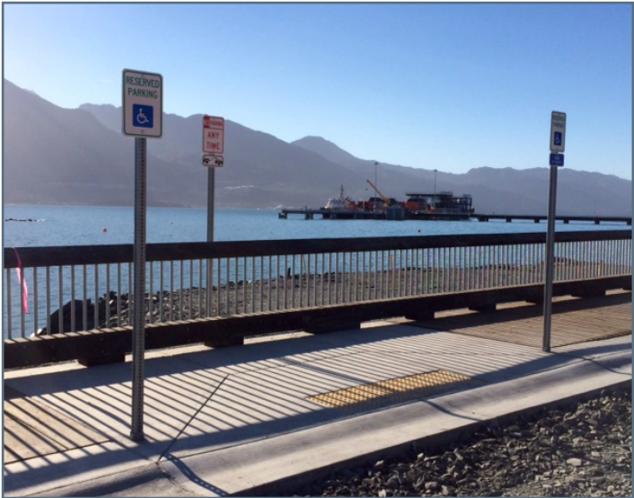
Sign posts grouted in holes drilled in the sidewalk
