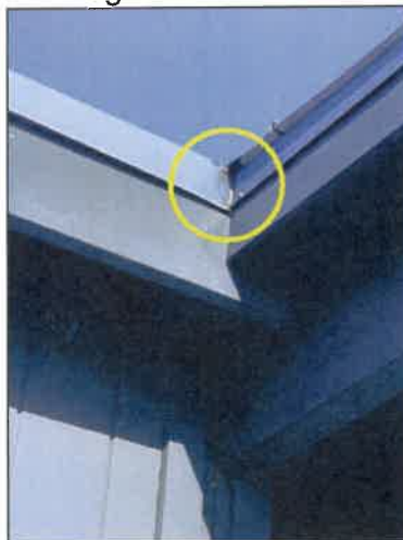
Recommend proper sealing for flashing.
