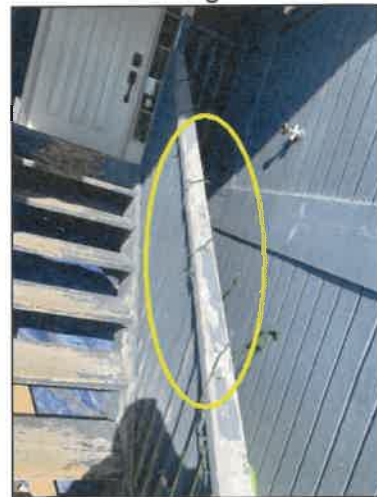
Handrail is not fully secure.
