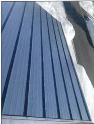
No fasteners on joining of ridge pieces. Loose screw.
