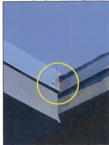
Recommend proper sealing of flashing.
