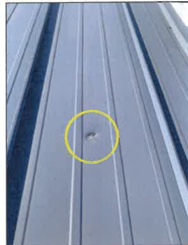
Dent with a small crack in the roof panel over the garage.
