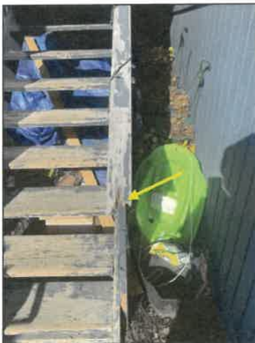
Handrail is damaged.
