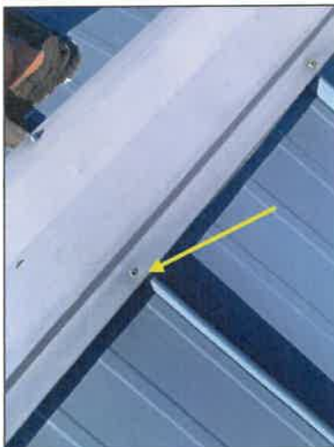
Missing screw on ridge.
