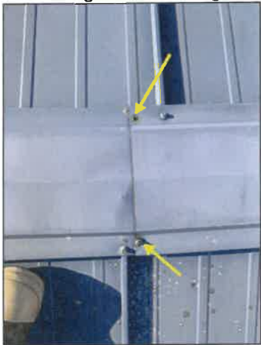
No fasteners on joining of ridge pieces. Loose screw.
