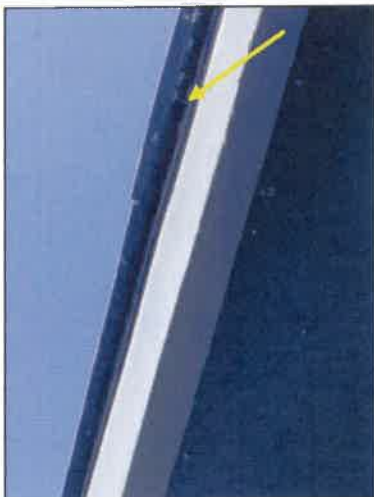
Screw causing drip edge to protrude.
