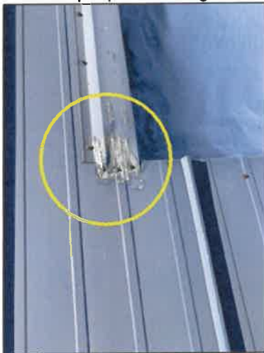
Recommend proper sealing for flashing.
