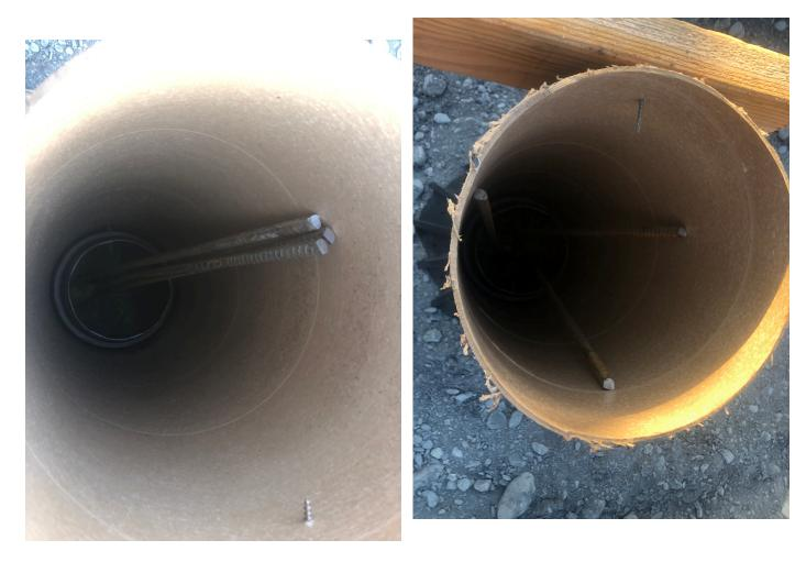
Photos taken prior to pour showing proper reinforcement. Note: Rebar is sitting on the ground in these photos. When the concrete is poured into the tube, the rebar is then lifted up to proper 3 inch height from the top of the tube.
