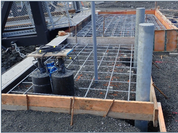
Rebar, arctic pipe risers, bollards for concrete slabs at bridge abutment
