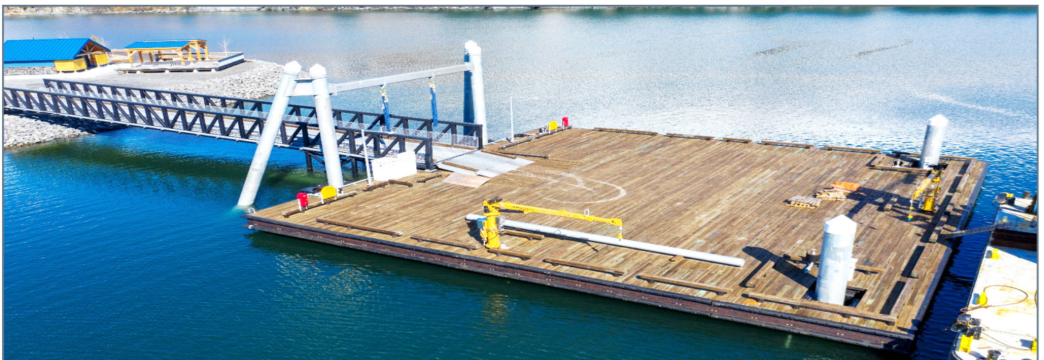
Transfer bridge (144' long) with steel grate deck, mooring frame and drive down float (90'x90') with timber deck and two 2-ton hydraulic cranes. Photo courtesy of J. Talbott.
