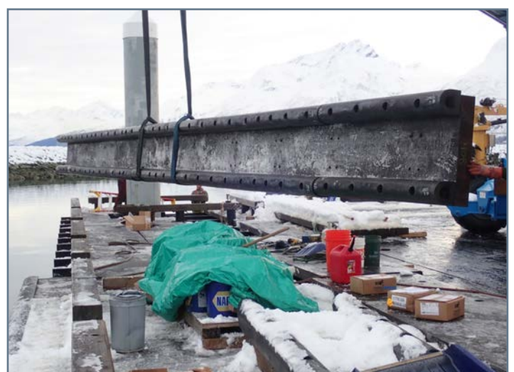
Installing fender assemblies on DD float
