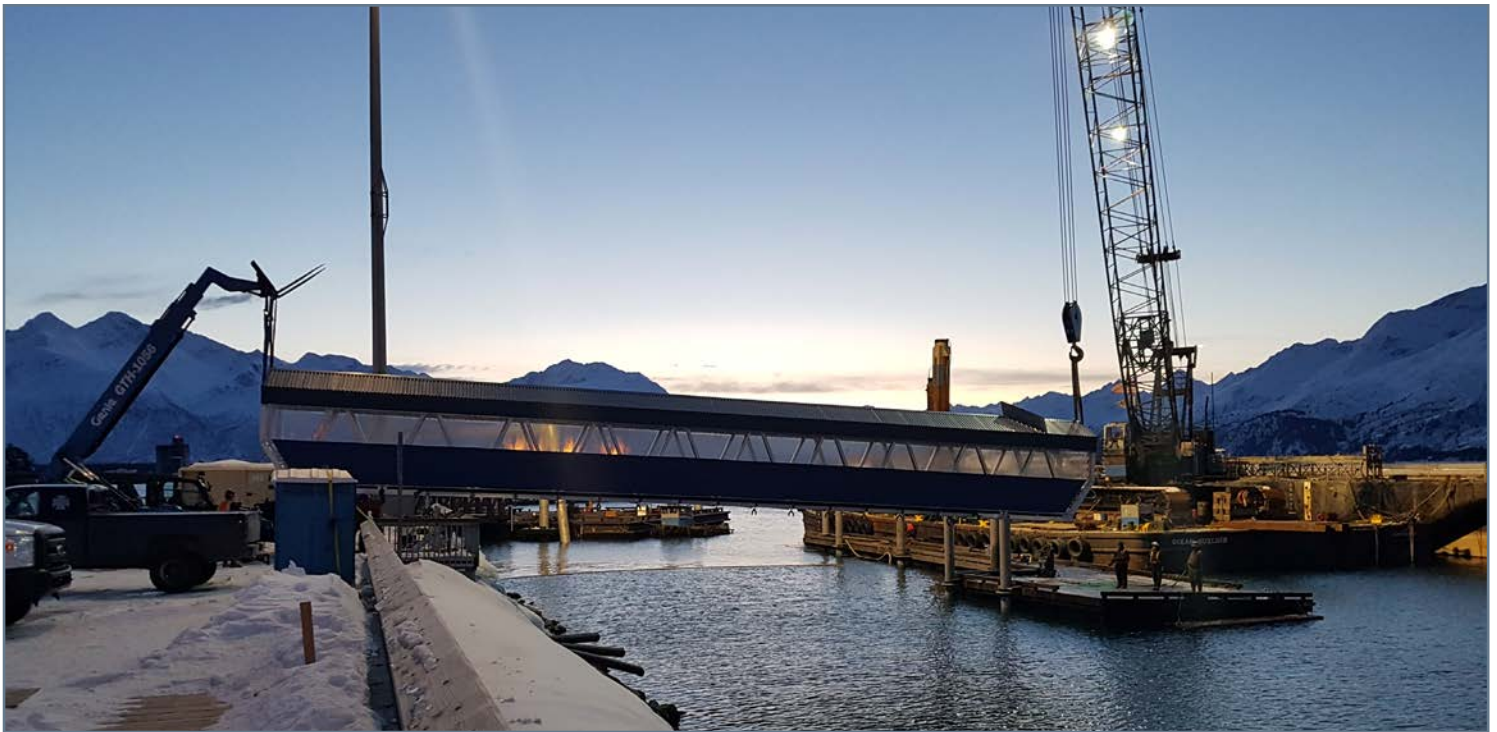
Lifting Gangway 3 into position on shore lug (left) and float landing plate
