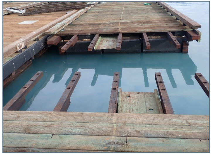
Head float stringers prior to overlapping, bolting and decking
