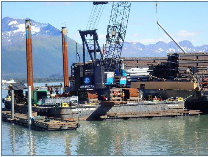
Crane lifting a pile from materials barge for installing on the west end of the head floats
