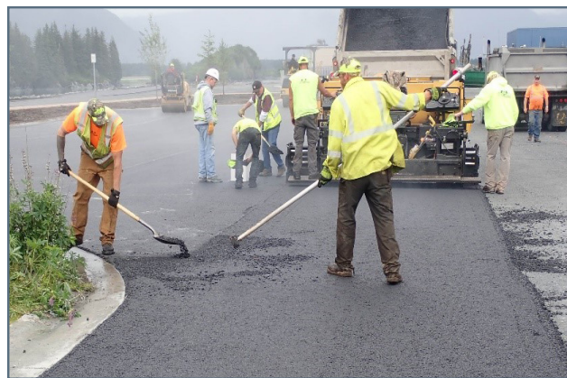
Spreading asphalt for parking area near Warehouse Building
