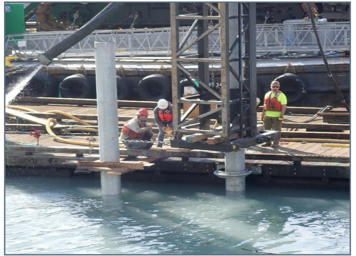
Temporary pile (left) maintains position of floats while drilling 10 feet into bedrock to install the first mooring pile for the head floats
