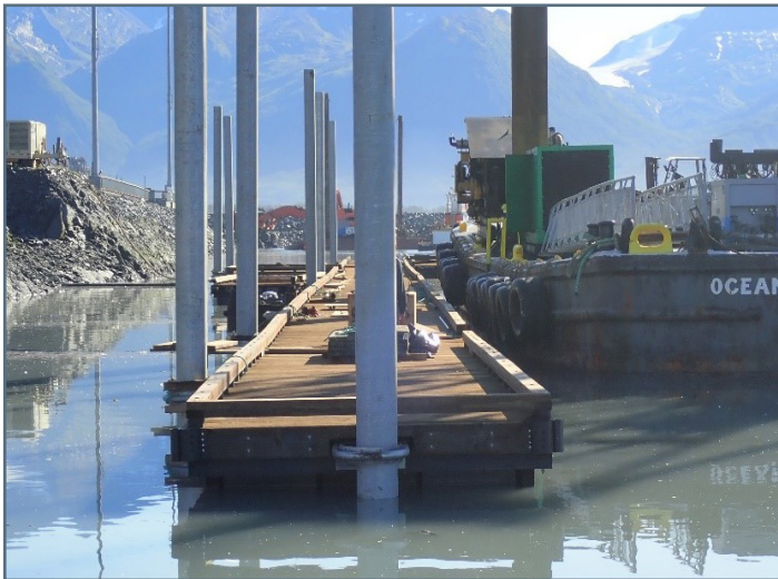
Piling installed for west portion of the head floats required drilling 10 feet into bedrock to create a "socket" for the piling
