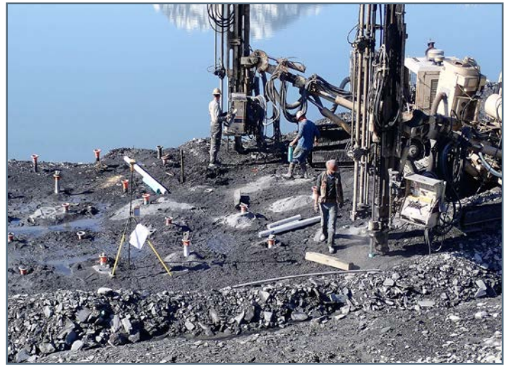
Drilling holes for blasting rock at the West part of mooring basin
