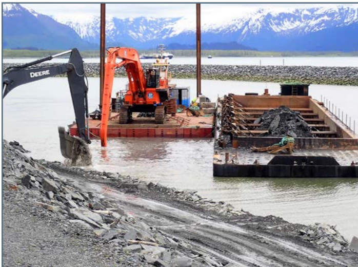
Deere 870 (at left) excavates and stages rock for EX1200 with clamshell bucket on Flexi-float barge to reach and place on dump barge
