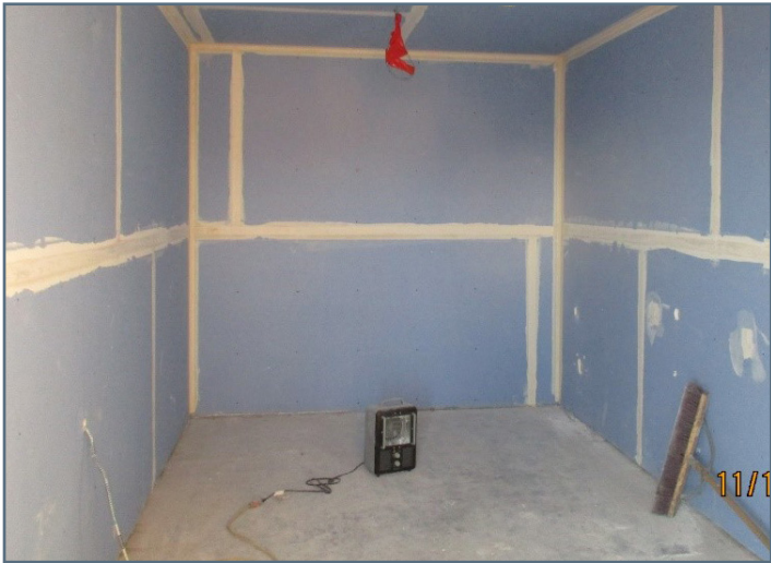
Restroom Bldg. - Taping sheetrock joints
