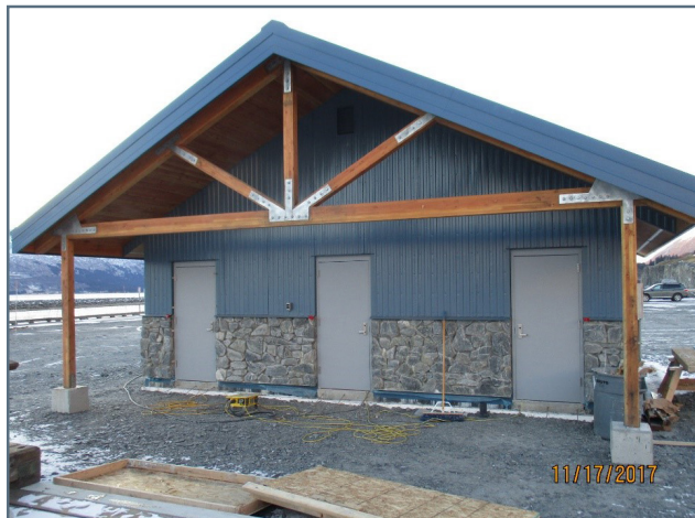
Restroom Bldg. – Glulam truss supports canopy
