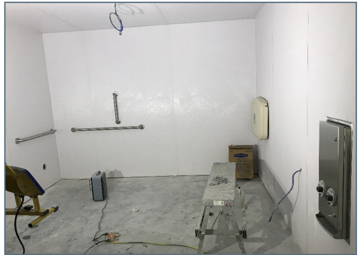
Restroom Bldg. - Grab bars and toilet accessories installed on FRP walls
