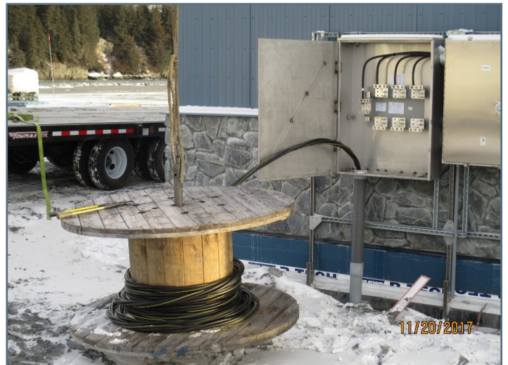
Bilge Bldg. - CVEA pulling wire from service panel to transformer
