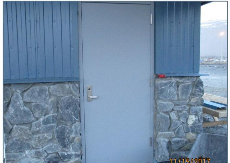
Restroom Bldg. – Fiberglass frame and door for Women restroom
