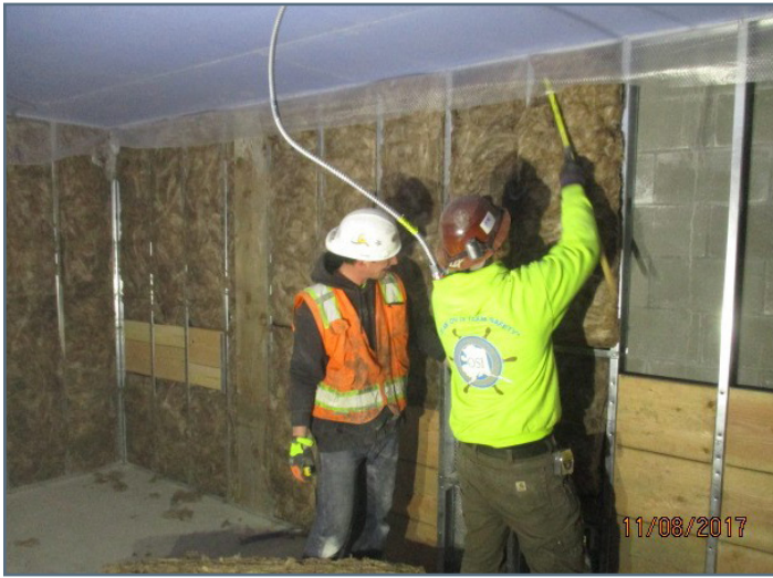
Restroom Bldg. - Installing batt insulation
