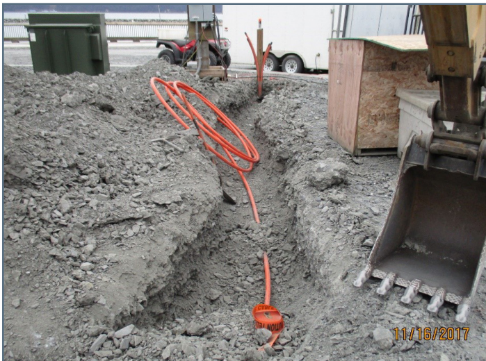
Bilge Bldg. - CVTC laying conduit for telecom service
