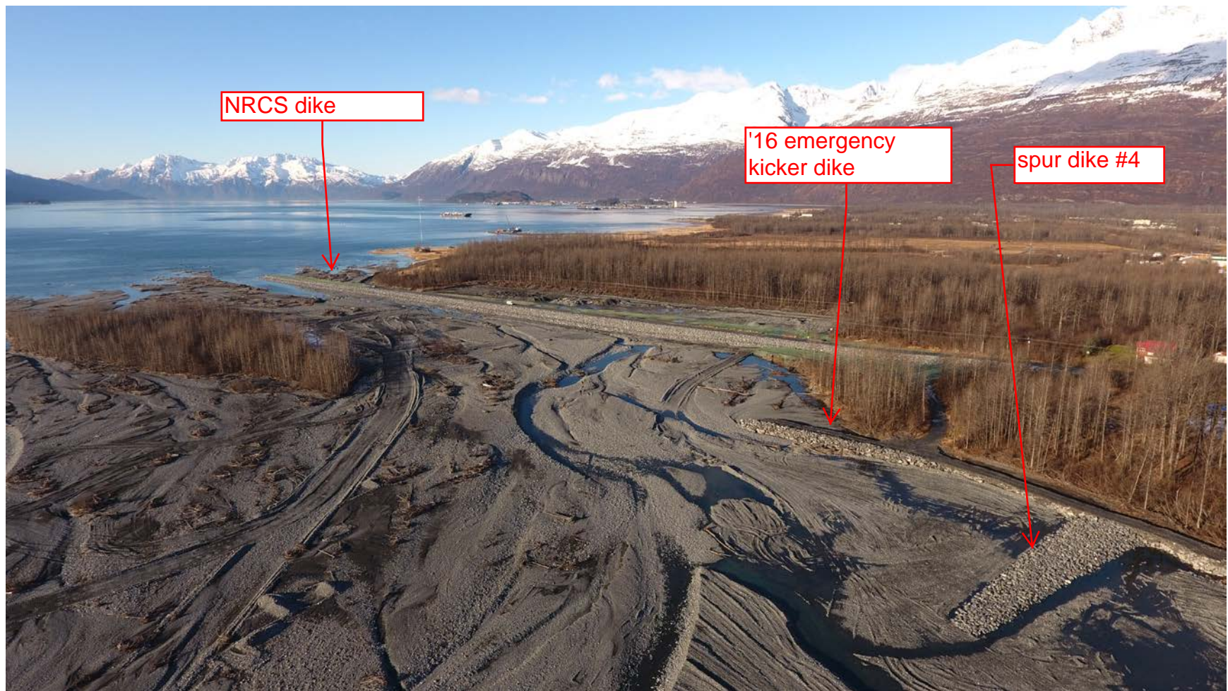
A low angle view of the dikes constructed to protect Copper Ave and the radio antenna the past two summers.
