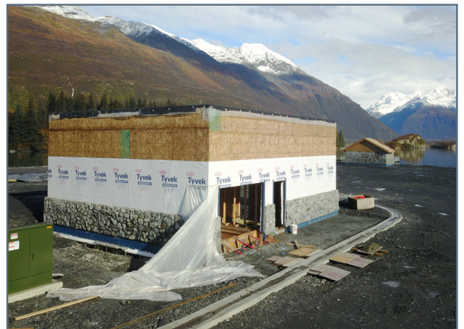
Bilge Bldg walls, stone veneer, roof installed; ready for siding
