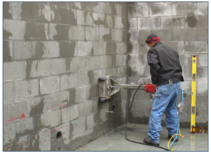
Restroom – Drilling Mechanical Room walls for plumbing pipe
