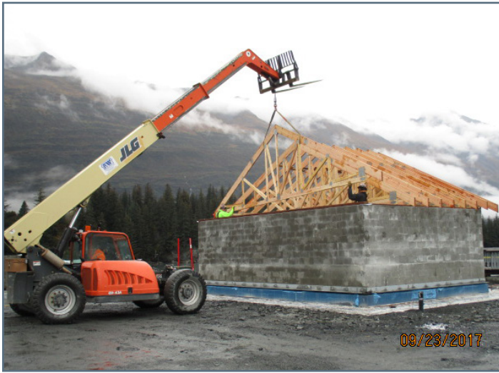
East Restroom – Setting roof trusses
