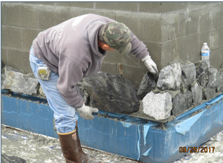
Restroom - Mortaring native rock wainscot on steel support
