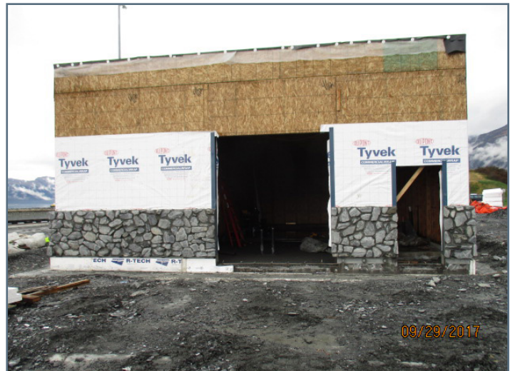
Bilge Building - Walls, stone veneer, roof installed; ready for siding
