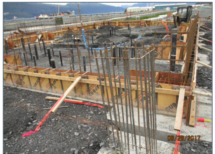
Warehouse Building - plumbing/electrical roughed-in, perimeter stem wall formed
