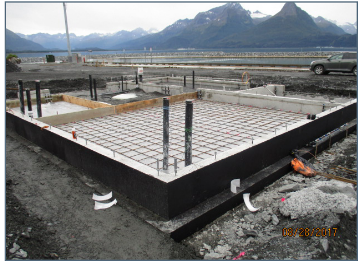
Bilgewater Treatment Building - footings waterproofed, prepared for slab
