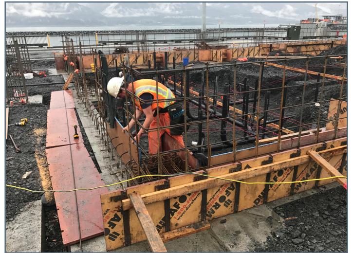
Warehouse Building - setting forms for perimeter stem wall
