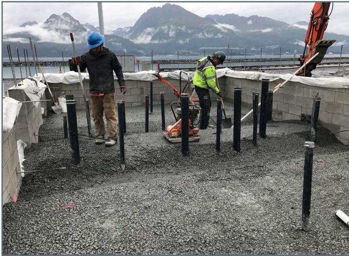
Restroom - backfill prepared for thickened slab at interior walls
