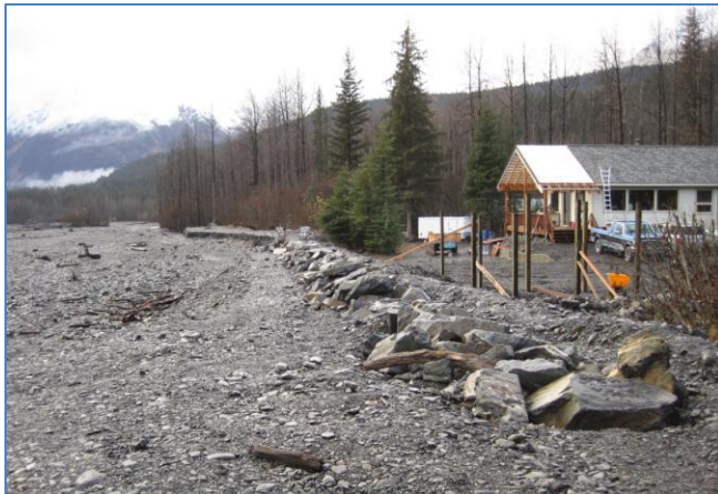
Photograph 3. Non-engineered levee with rock placed by homeowner in the Questa Woods subdivision (looking downstream)
