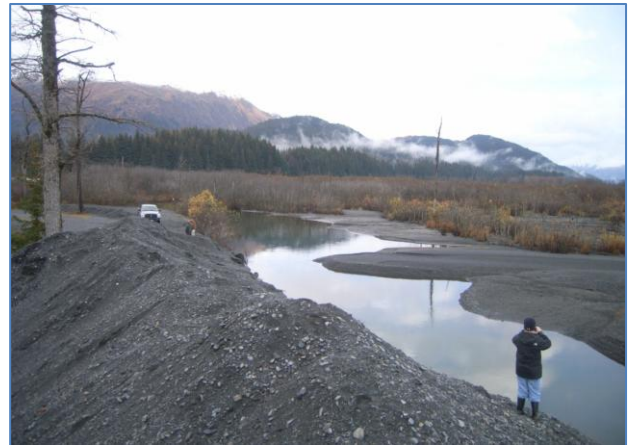
Photograph 4. Embankment constructed of river-run materials along Clear Creek near Salmon Creek confluence (looking upstream)
