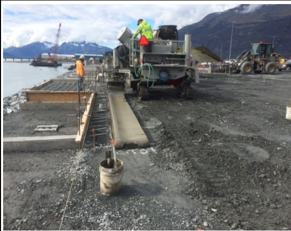
Machine placing curb & gutter at maintenance pad
