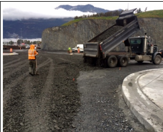
Delivering Type II-A gravel for final subgrade
