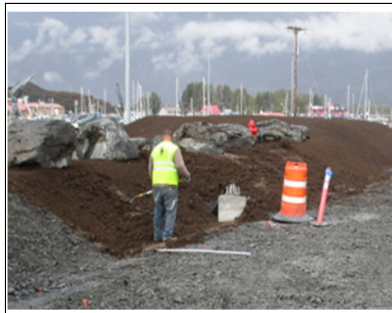
Spreading topsoil on berm along West Access
