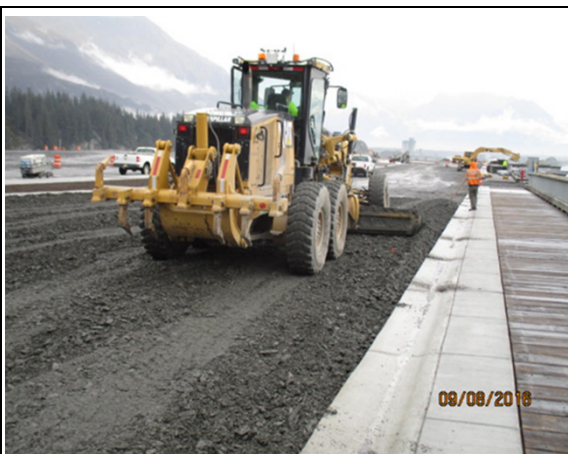
Grading Type II-A to proper elevation along curb
