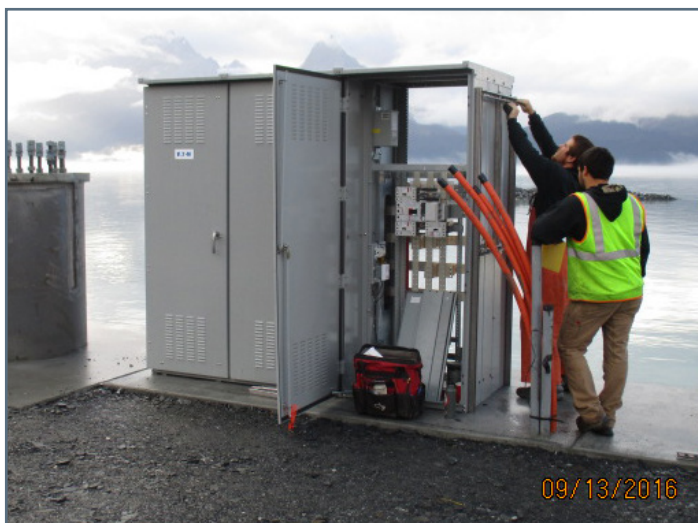
Installing cabinet for electrical distribution to floats
