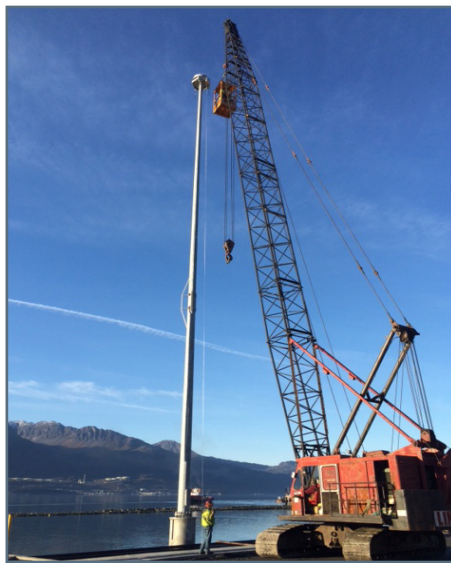
Crane setting 100-foot high mast light pole on foundation
