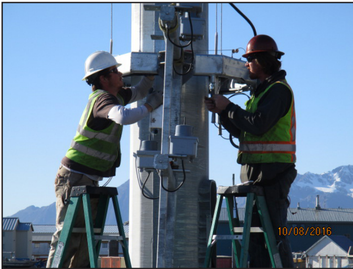
Installing high mast light fixture array
