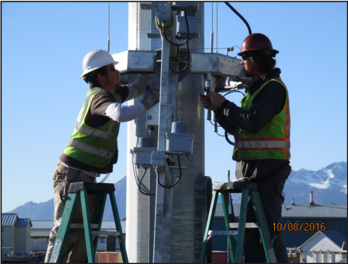
Installing high mast light fixture array
