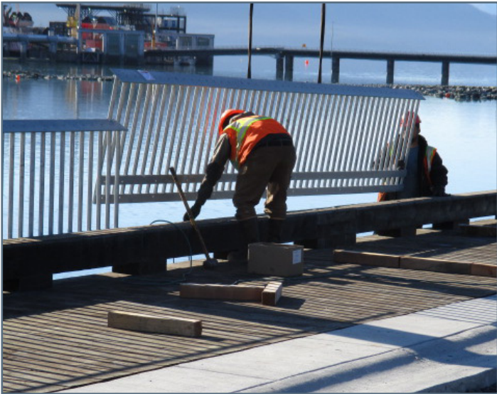
Placing guardrail for the boardwalk
