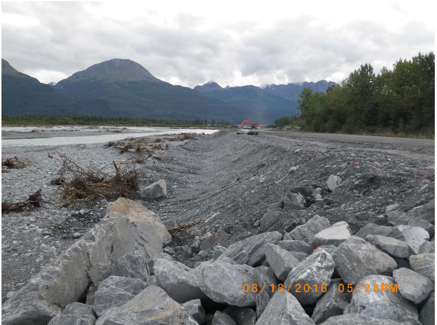
After photo, looking towards bridge. The bank has been sloped and riprap has been placed in the foreground.
