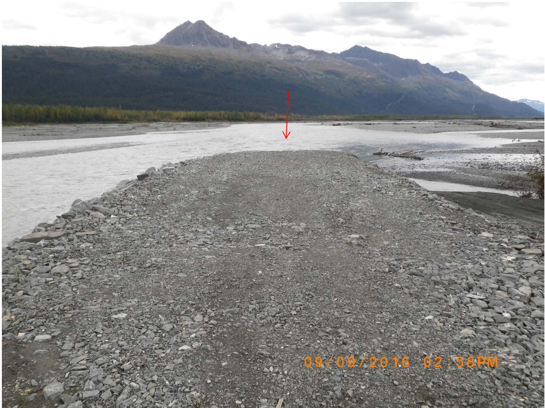
A 19' wide by 52' long extension was constructed off the end of groin #1.
