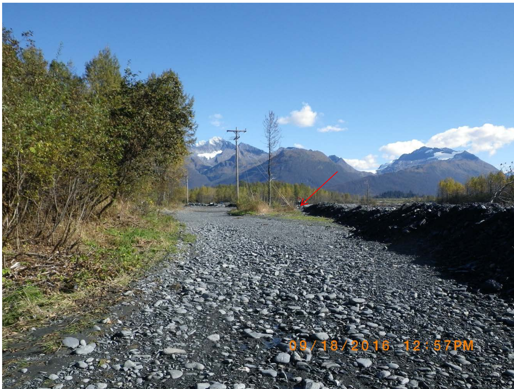
Looking upstream on Copper where the flood waters stripped away the topping material from the roadway. Note the proximity of the guy wire to the river bank.
