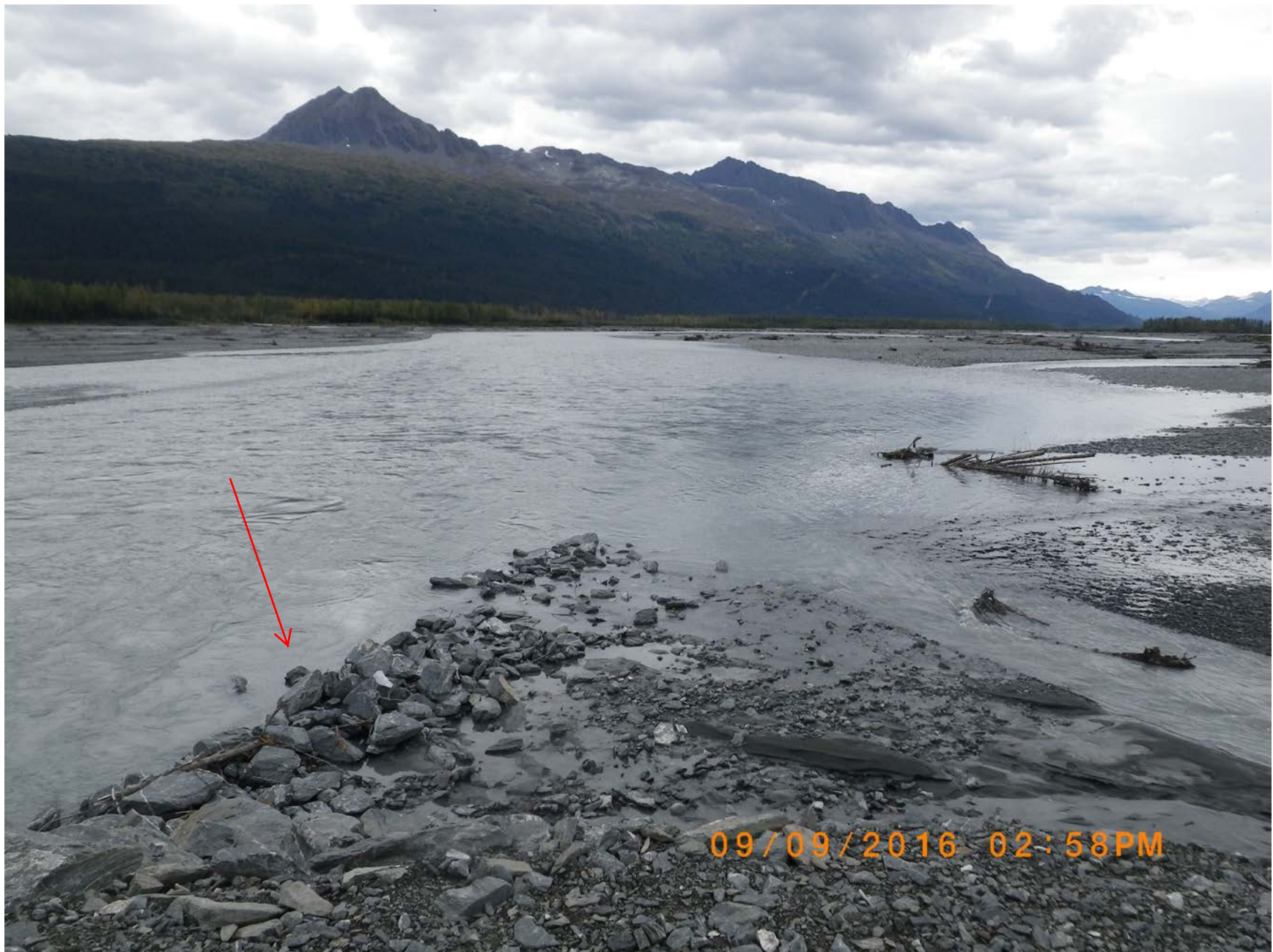
A 32' long rock spur dike was constructed off the end of Groin #1.
