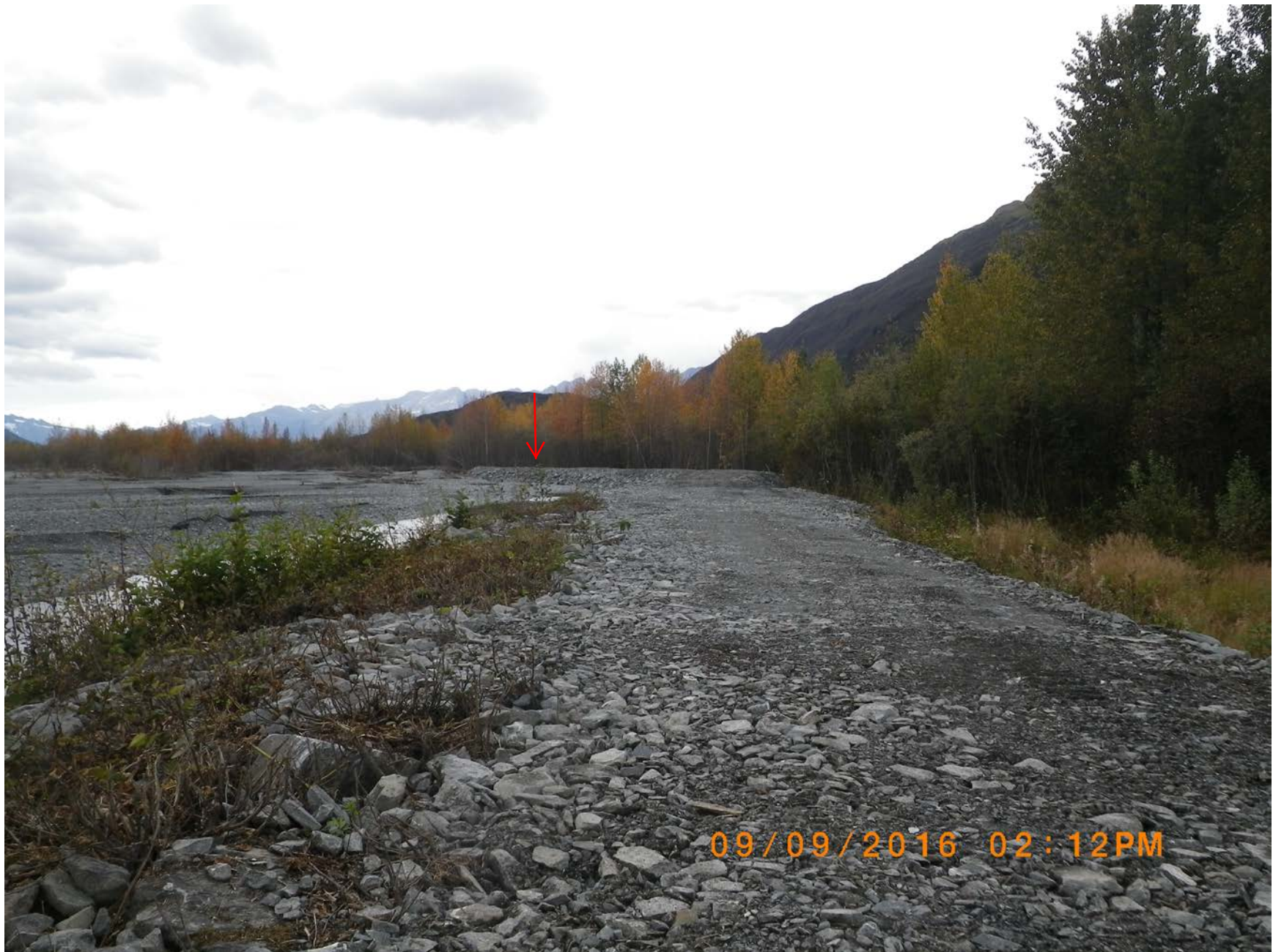
Groin #4 at low water. This section of dike was extended last summer and again this summer. Approximately 347' of new dike was constructed this year of the end of groin #4. It is approximately 13' wide at the top.
