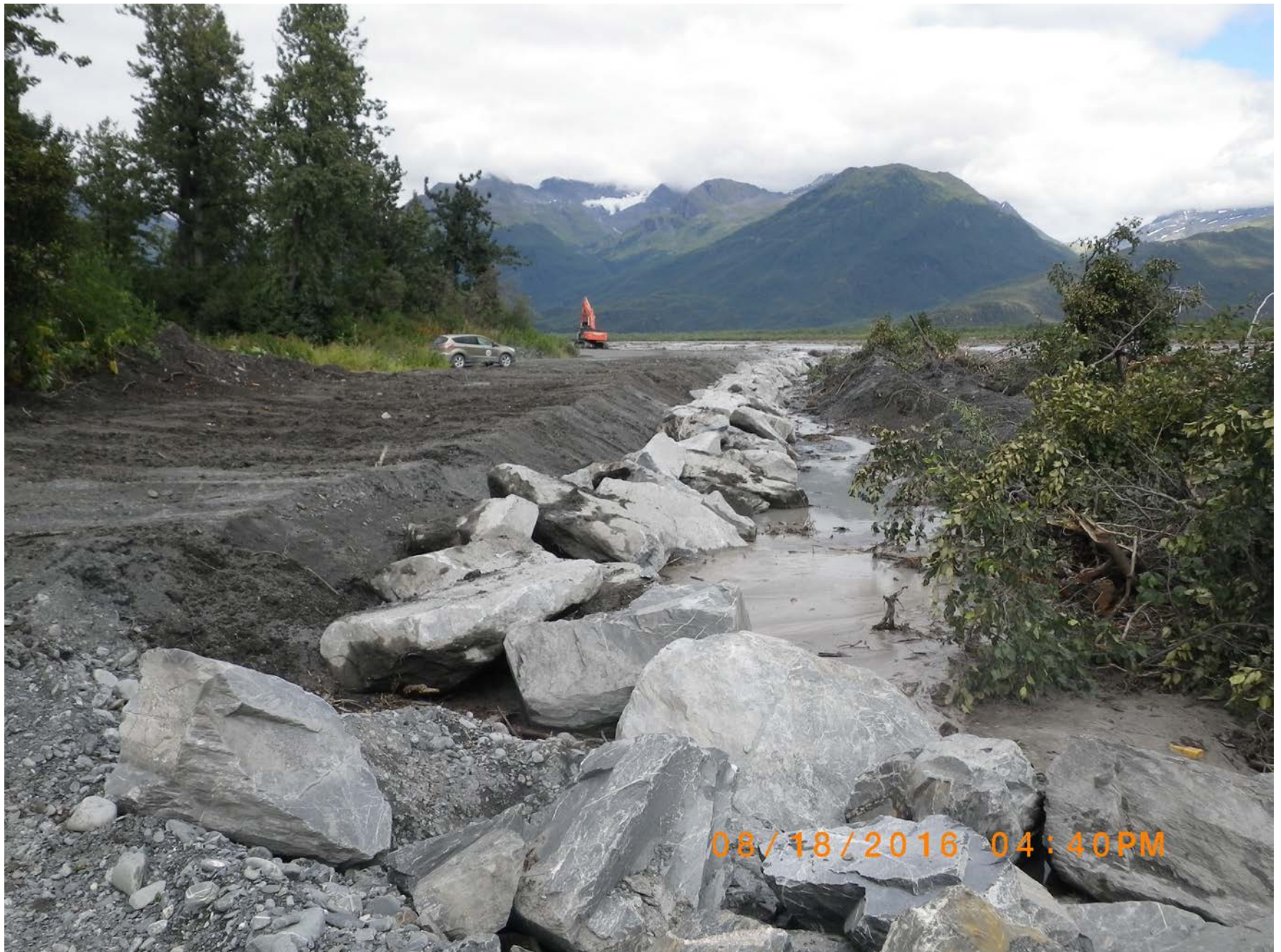
Looking upstream at the end of the project. Large rock actively being placed.
