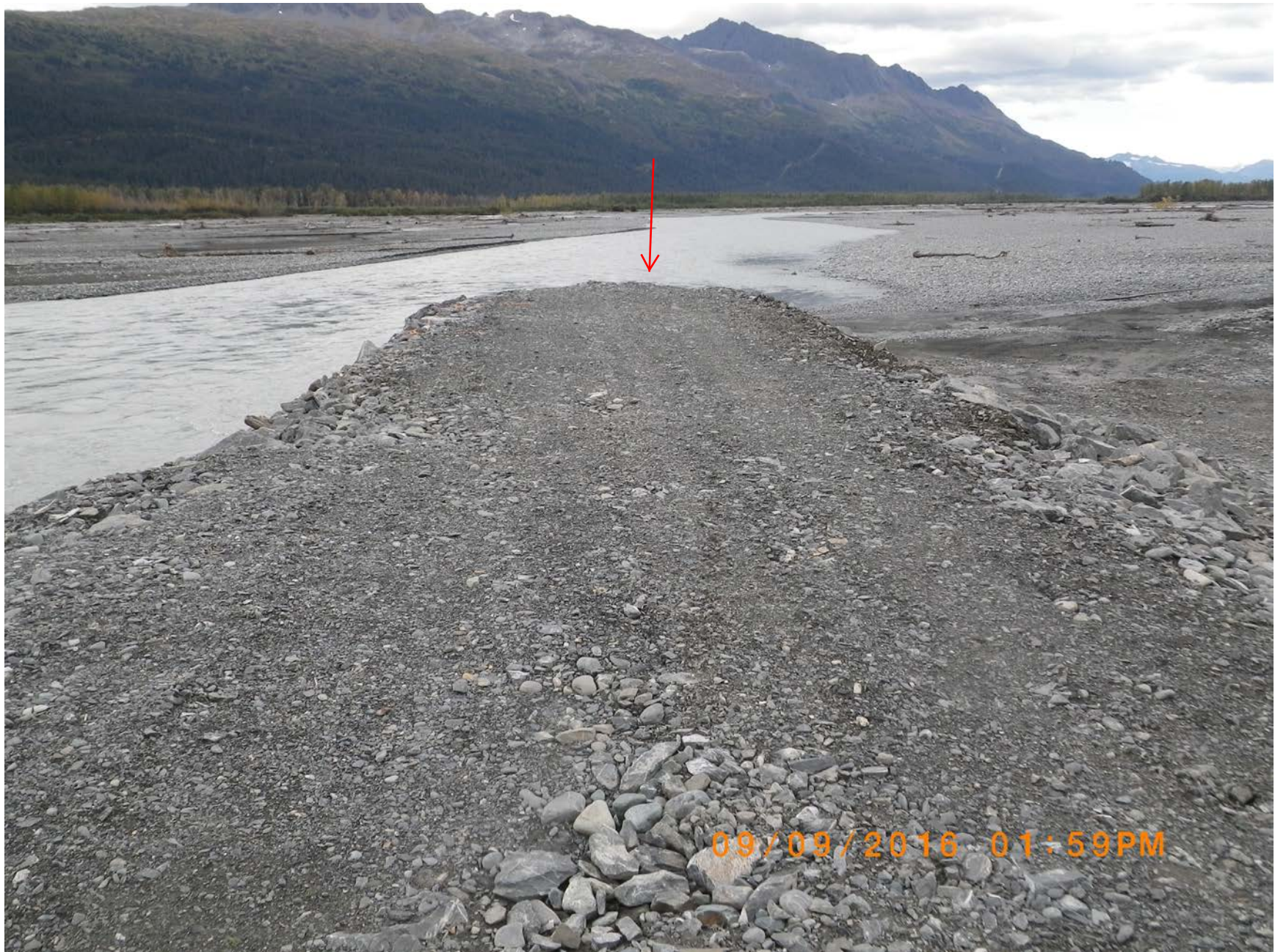
Groin #2 extension - The existing groin was extended out into the river. The new structure measures 18' wide at the top and 70' long.
