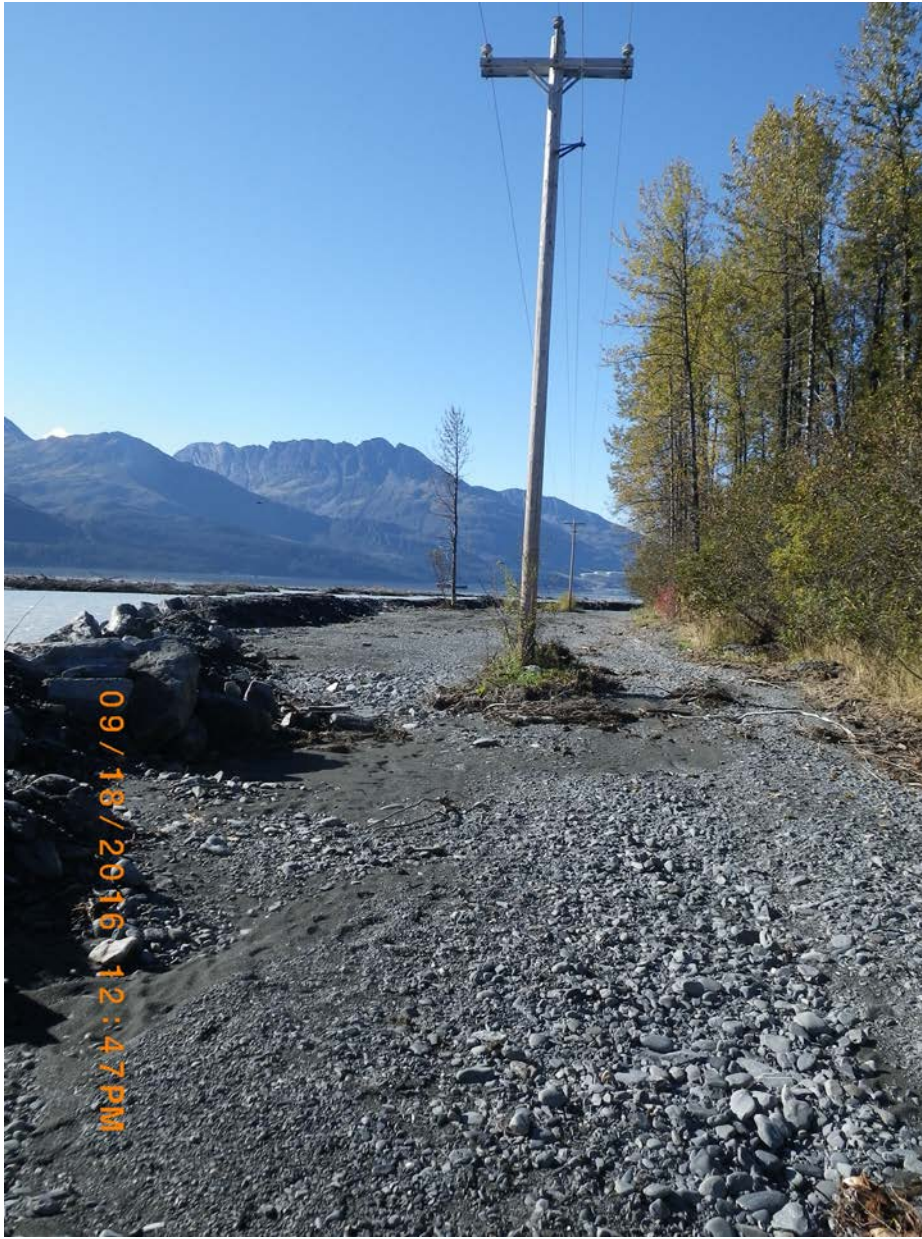
Flood damaged roadway and the proximity of the river to the electrical utilities.
