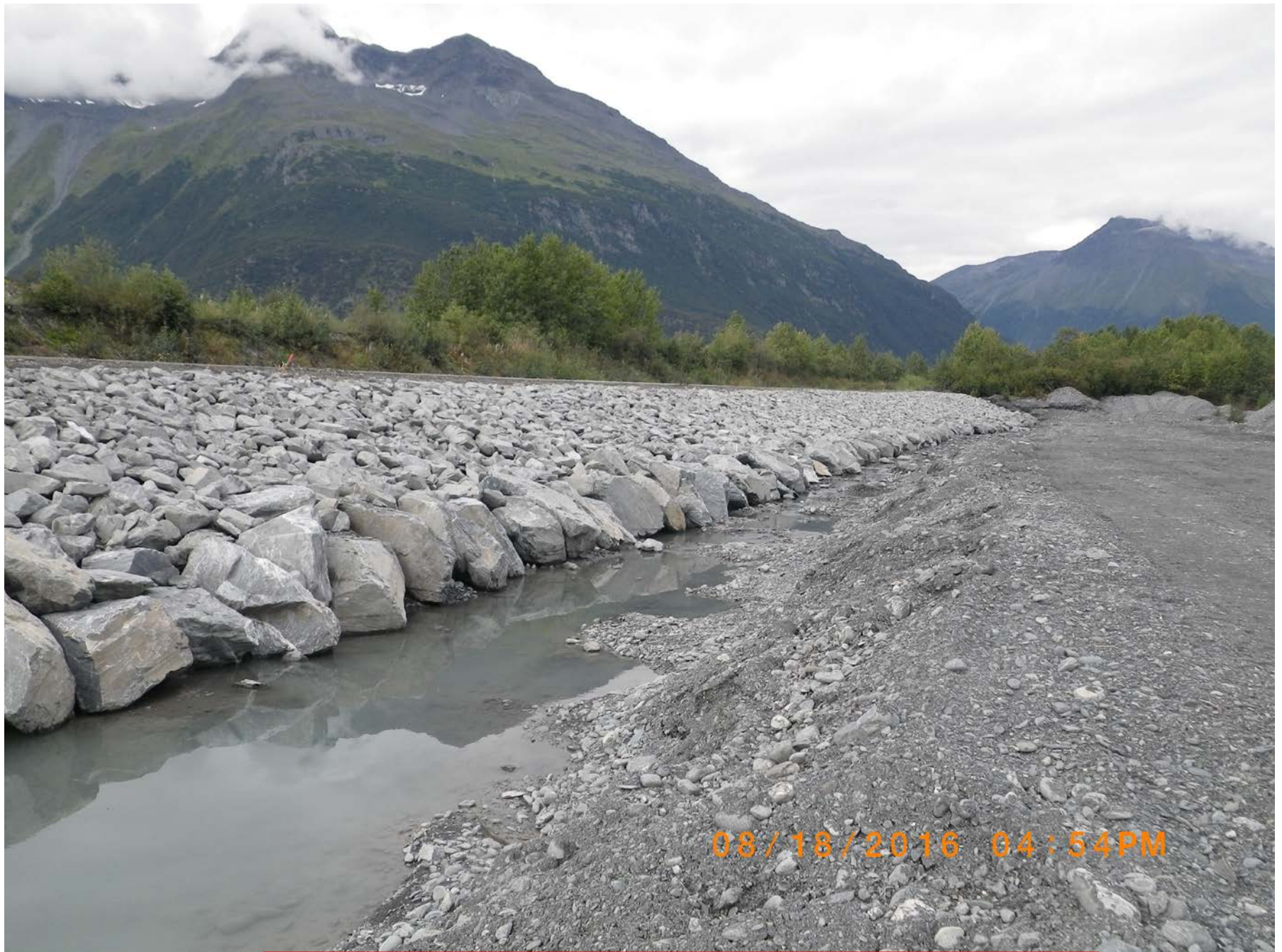
View from the river bed of the newly armored slope near the beginning of the project.
