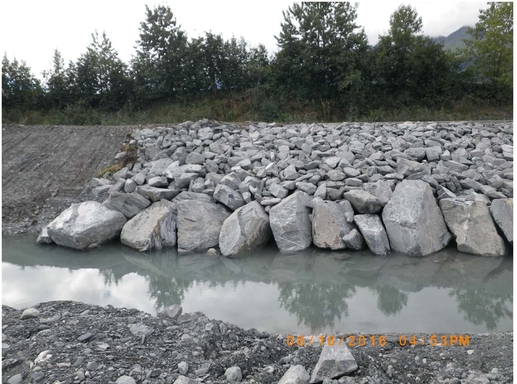
View from the river bed of the newly installed riprap on the sloped bank. Riprap work has been completed since this photo was taken.
