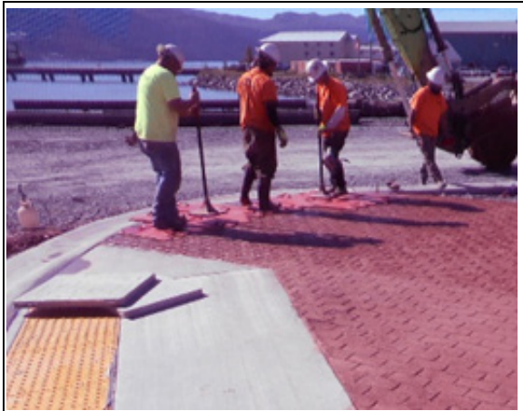
Stamping brick pattern into red concrete
