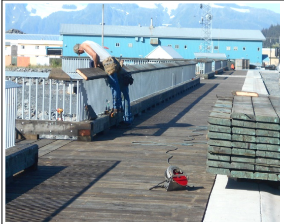
Attaching timber top plate to guardrail assembly
