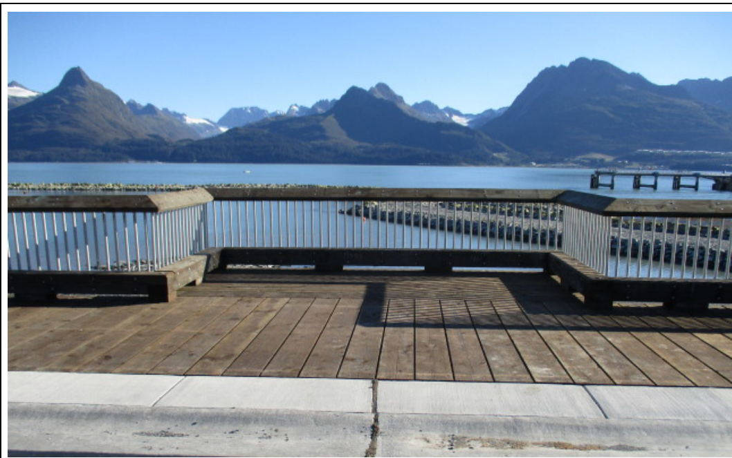
Concrete curb and sidewalk, boardwalk decking, bullrail and handrail at West Rest Area
