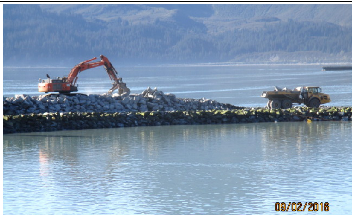
Western Marine truck delivering armor rock for excavator to place near entrance end of south breakwater
