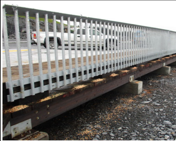
Boardwalk guardrail attached at bottom to bullrail
