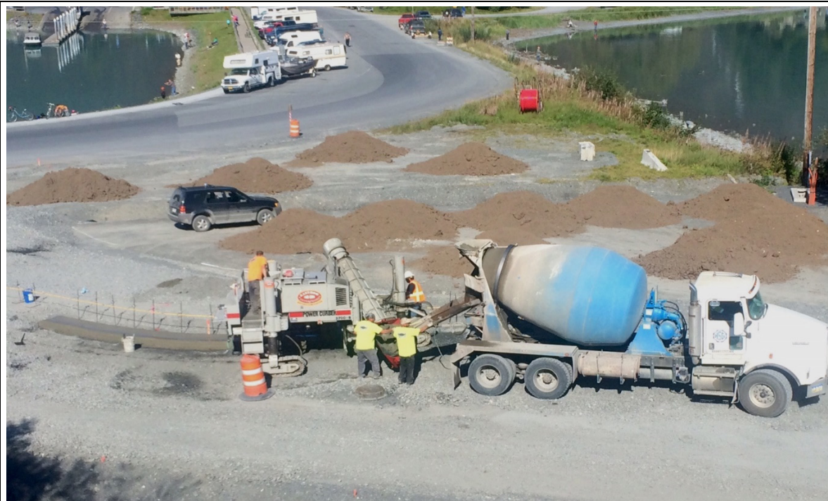
Slipform machine placing curb and gutter along East Access; topsoil stockpiled for spreading near entrance
