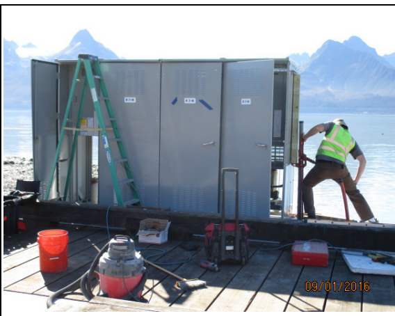
Setting cabinet for main meter and east Ramp #3
