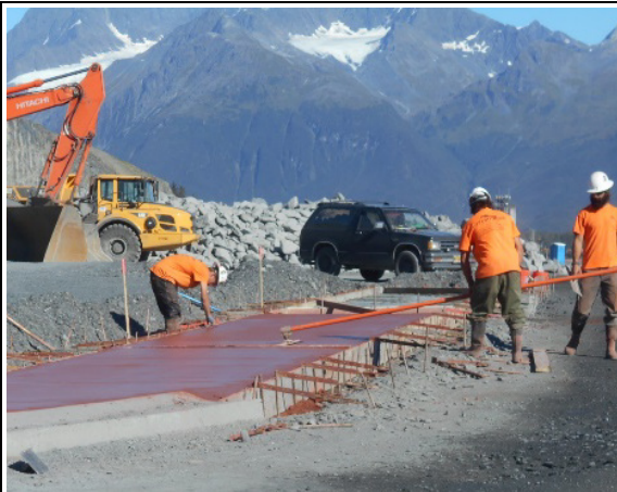
Finishing concrete for sidewalk prior to stamping
