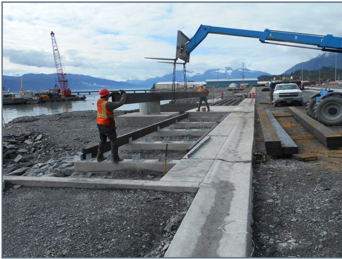
Setting glulam beams in brackets attached to concrete sleepers
