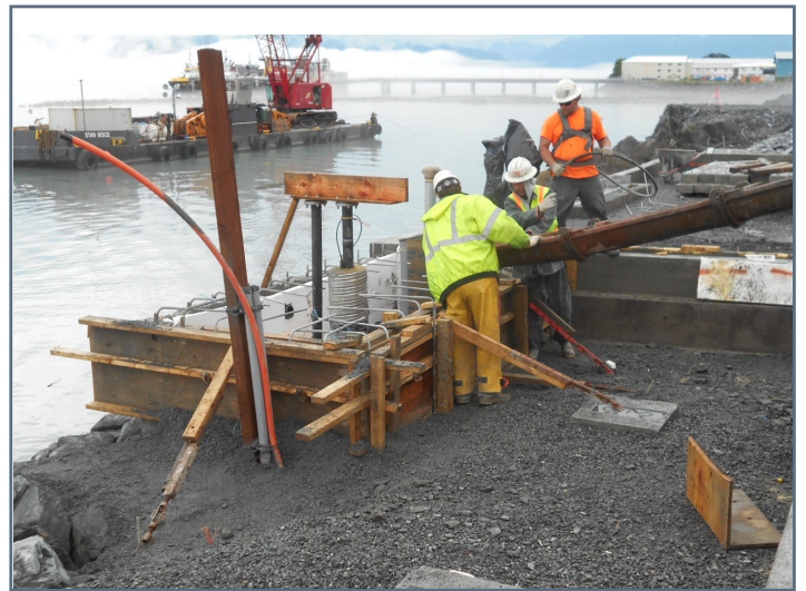
Placing slurry backfill around utility stubups before placing the concrete slab
