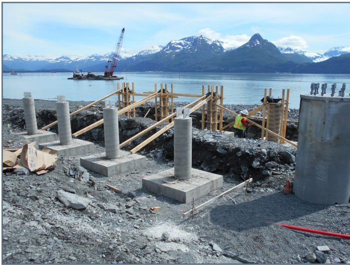
Removing forms at columns to support canopy for future picnic area; high mast light foundation (at right)
