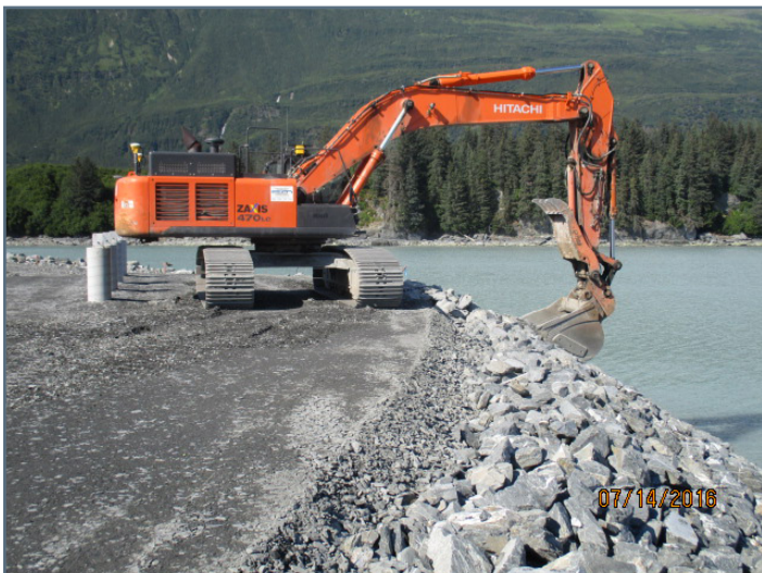
Placing riprap on the fill slope near the east picnic area
