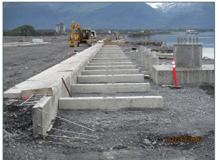
Concrete curb and sidewalk (left), boardwalk sleepers (center), high mast light base (right)
