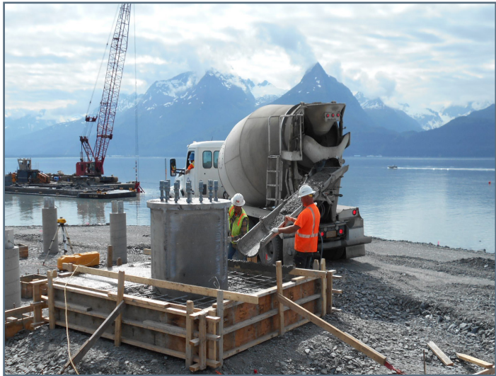
Placing concrete for pad around foundation piling for high mast light pole
