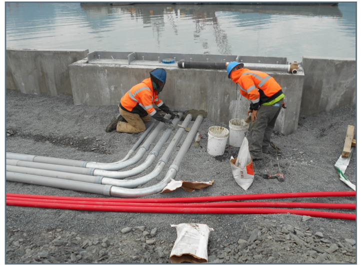
Grouting conduit penetrations at ramp abutment for utility services to the floats
