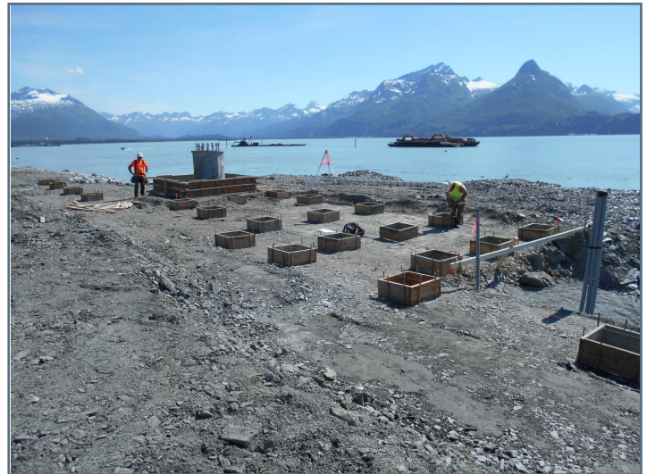
Forming pads for sleepers that will support the wood beams and deck for west picnic area
