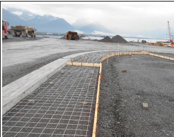
Mesh on concrete blocks for island area sidewalk
