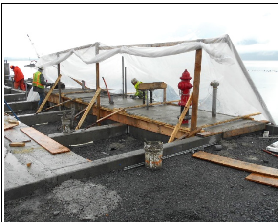
Plastic protects concrete finishing at utility slab
