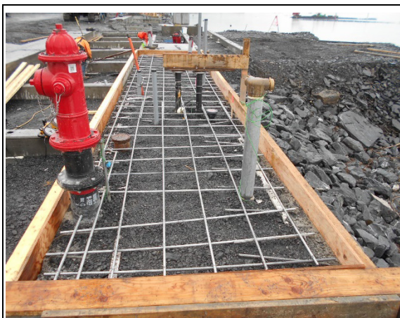
Steel mesh and forms at utility slab
