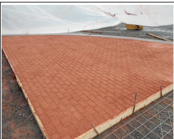
Brick pattern imprinted on concrete at island area
