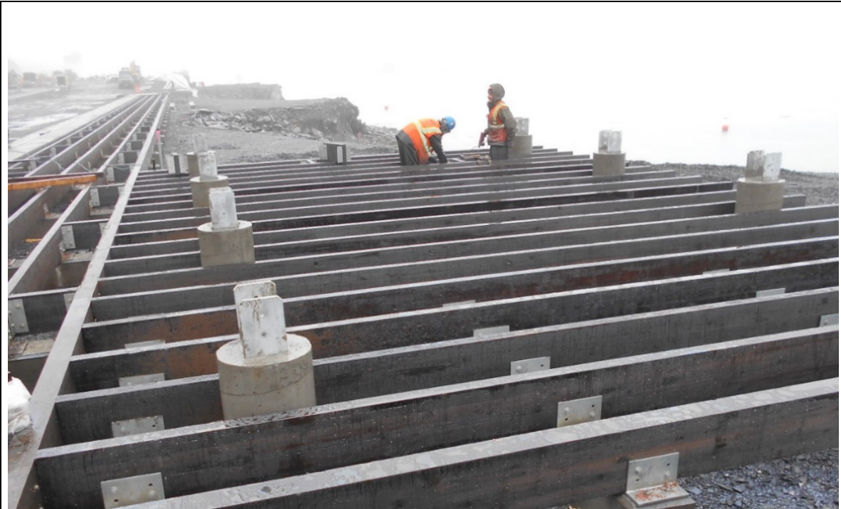
Glulams for West Picnic Area have been placed and secured with saddle brackets. Steel brackets on top of the round concrete pilings will support the canopy structure (part of future building contract)
