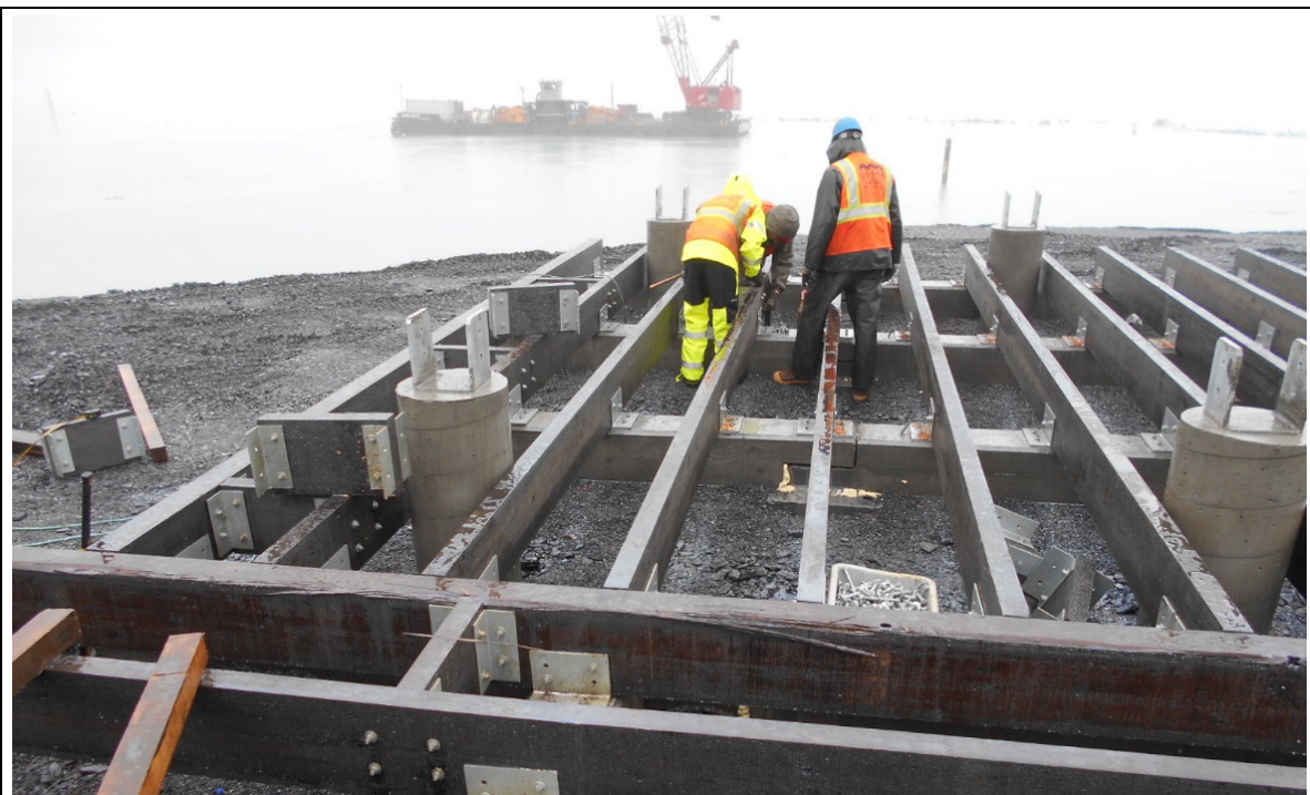
Installing solid blocking between glulam beams for the West Picnic Area
