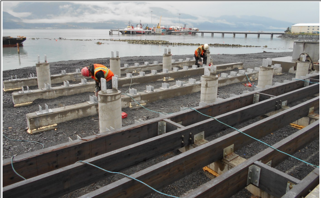
Installing saddle brackets on picnic area sleepers to secure glulam beams (like boardwalk beams at bottom right)
