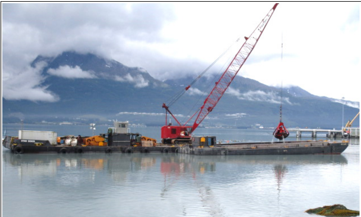
Western Marine continues dredging sediment to create the maneuvering channel and basin for the new harbor
