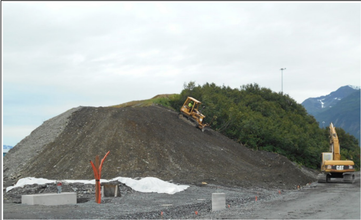
The slope at the east end of Hotel Hill was final graded for seeding
