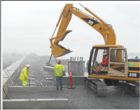
Placing precast concrete sleepers for boardwalk
