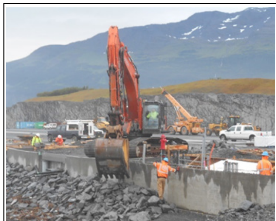
Placing riprap to protect abutment at Ramp #1
