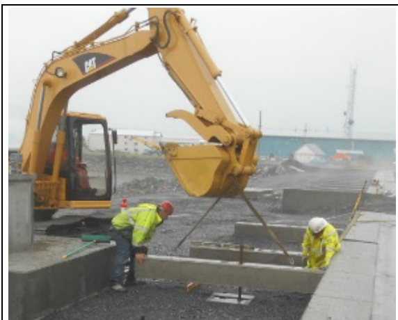
Aligning sleepers on top of concrete pads
