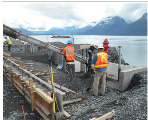
Backfilling BFP foundation with cement slurry
