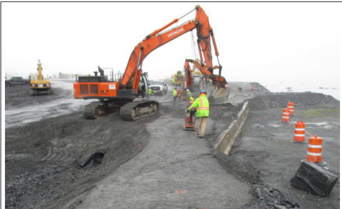
Compacting fill for a berm between the West Access and barricades placed along SERVS property
