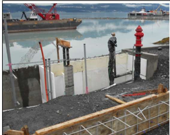
Insulating backflow preventer (BFP) foundation
