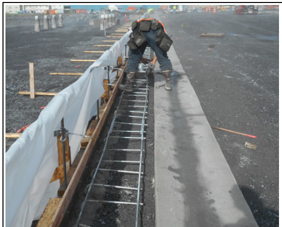
Tying rebar between boardwalk stemwall and curb
