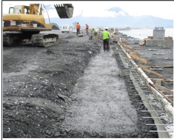
Compacting subgrade for curb along boardwalk
