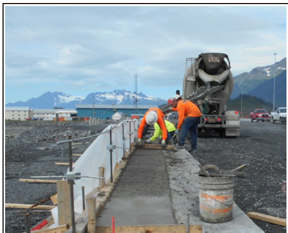
Finishing fresh concrete between stemwall and curb
