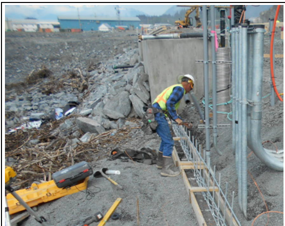
Placing footing rebar for utility pad wall
