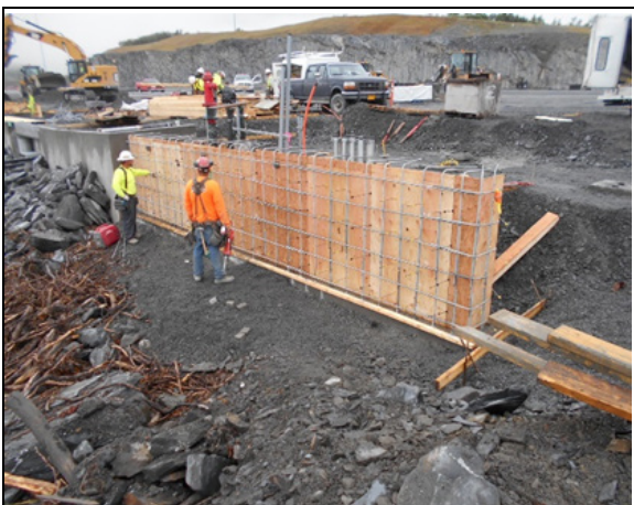
Placing forms and rebar for utility pad wall
