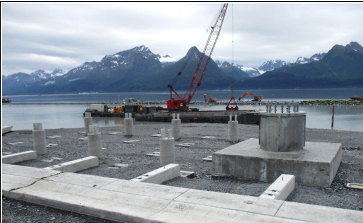
West Picnic area canopy post foundations and deck sleeper keys (center left); high mast light pole foundation (center right), boardwalk sleepers, narrow sidewalk and curb (bottom)
