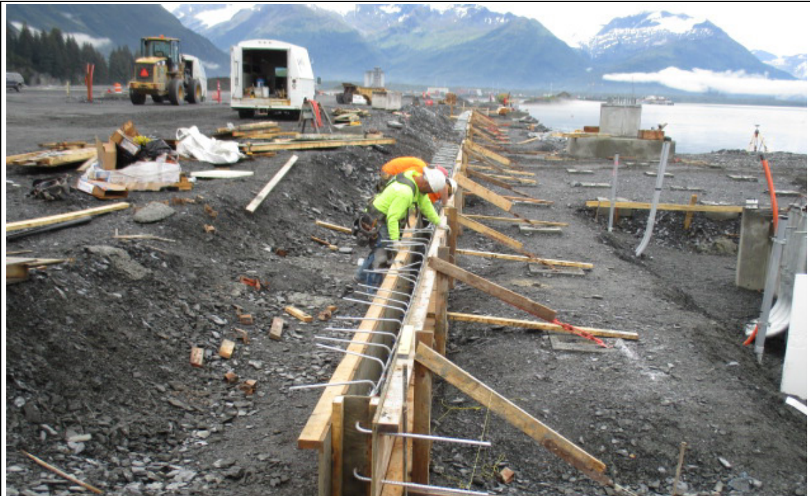
Continuing to place forms for stemwall between curb and narrow sidewalk (left) and boardwalk (right)
