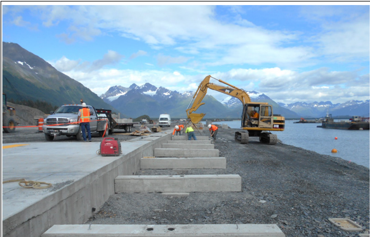
Placing pre-cast concrete sleepers on cast-in-place keys, which support timber beams and decking for boardwalk
