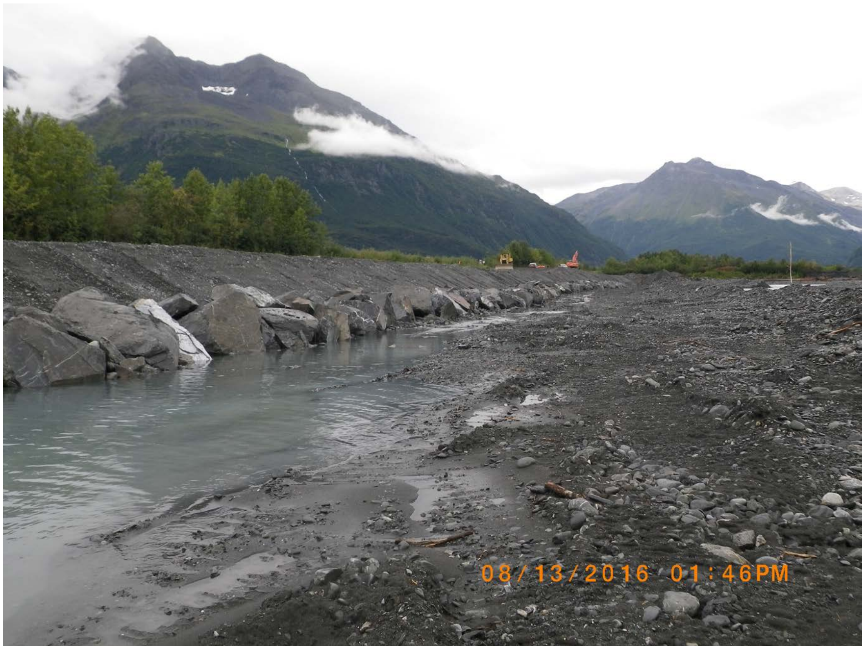
Looking back towards BOP with class 5 riprap placed at the toe of the slope.
