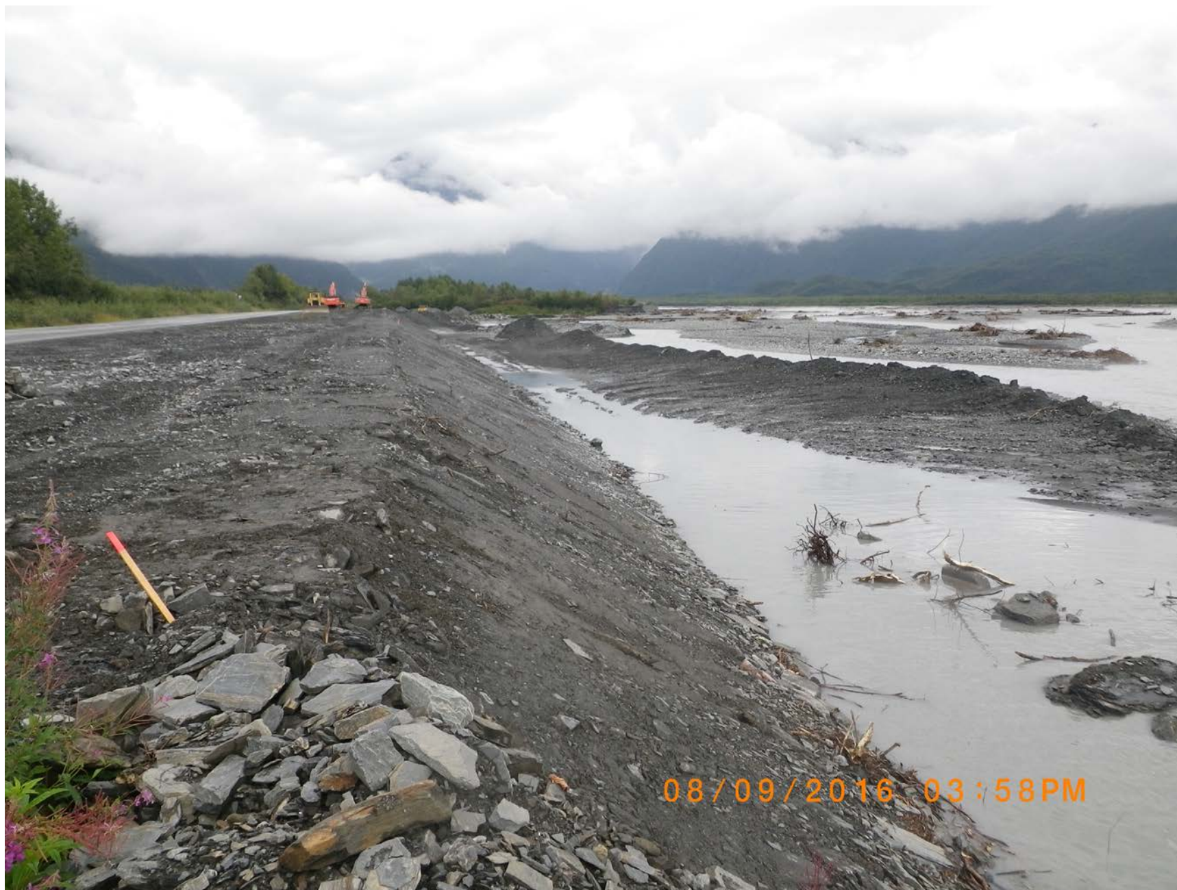
Looking back towards BOP. The contractor constructed a gravel berm to keep the flowing water out of the work area.
