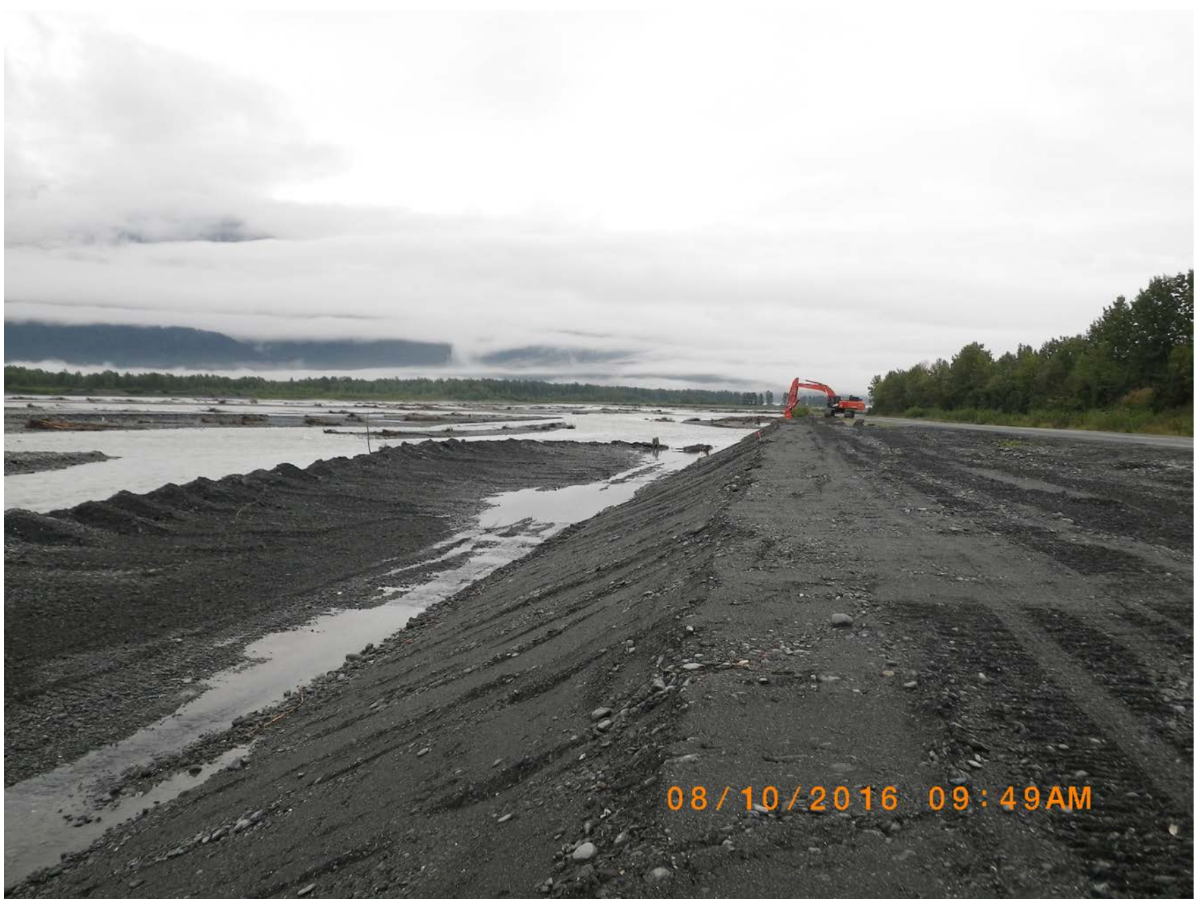
Looking towards bridge as the Hitachi 470 excavator works to slope the existing bank.
