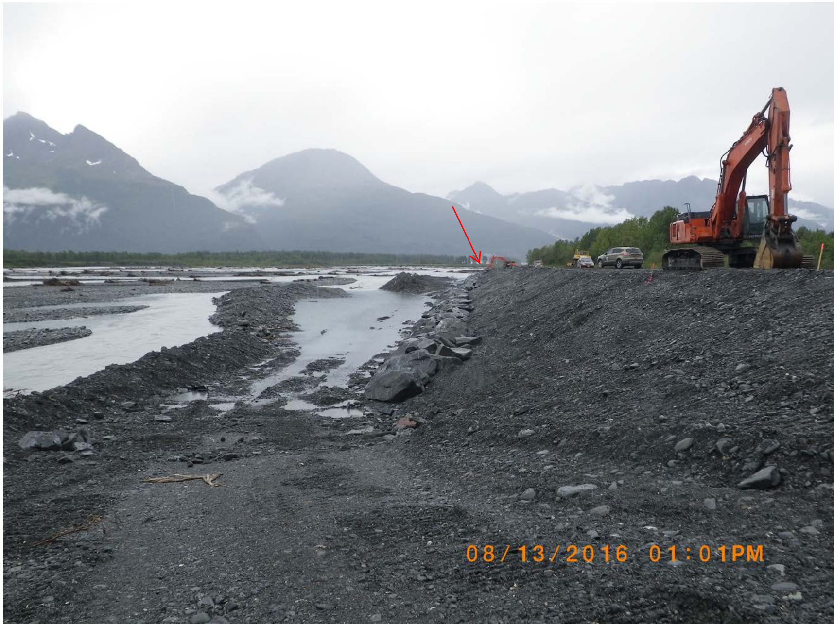
Looking towards bridge, the Hitachi 470 excavator working to place class 3 riprap.
