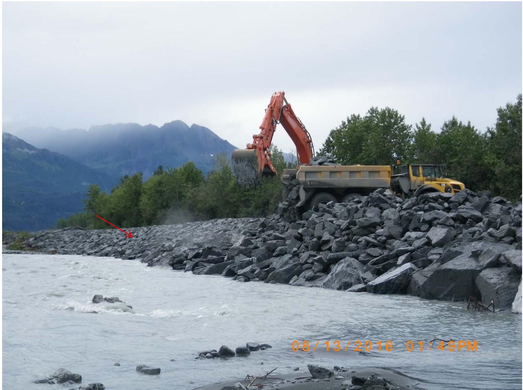
A rock truck delivers a load of class 3 riprap. The excavator has placed and sloped the class 3 riprap at 3:1.
