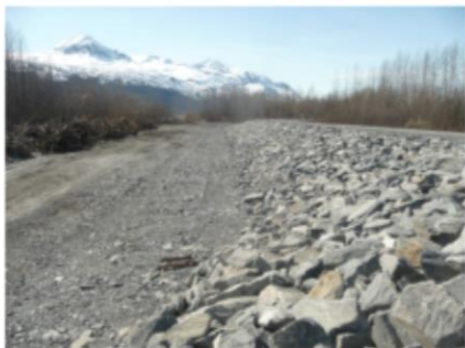
Completed Section (Scour Toe Buried)
