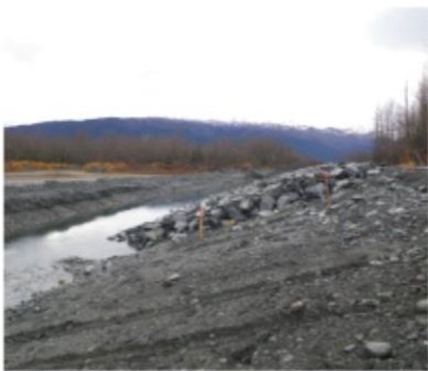
Trenching for Buried Scour Toe
