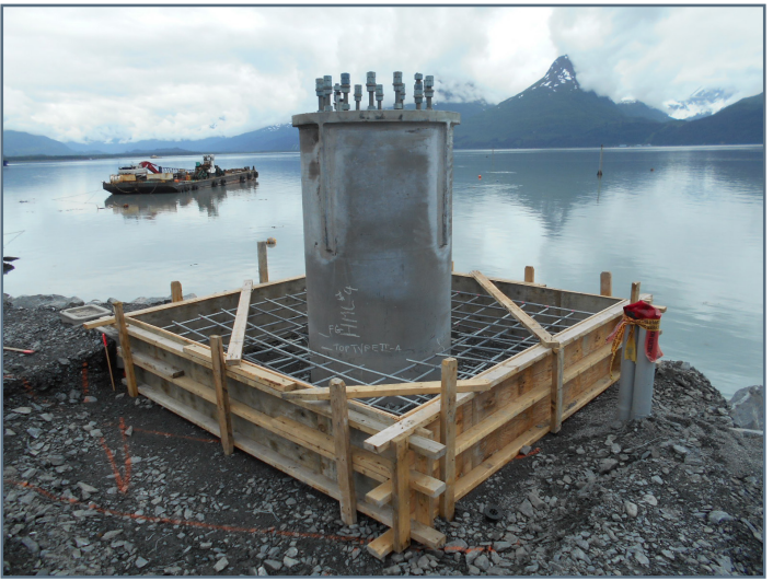
Form and rebar for concrete slab around high mast light foundation
