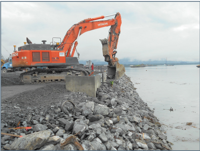
Placing riprap on slope at retaining wall for ramp
