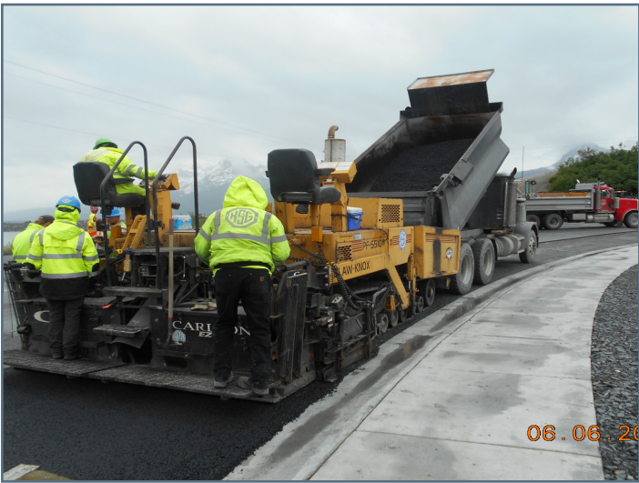
Paving between existing road and new curb & gutter
