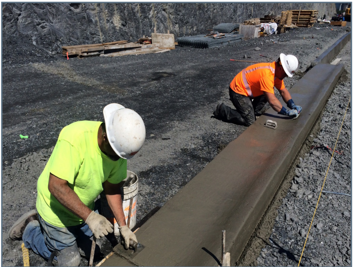
Cutting contraction joint and hand finishing curb and gutter
