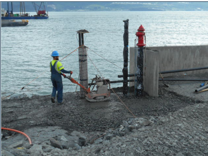
Compacting fill around water system risers and fire hydrant near ramp
