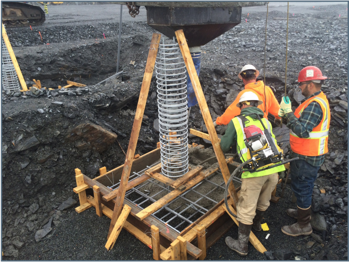
Placing concrete for base of pier to support picnic area canopy
