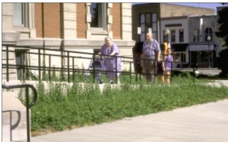
A historic town building added a ramp, walkway, and modified an entrance to provide access.
