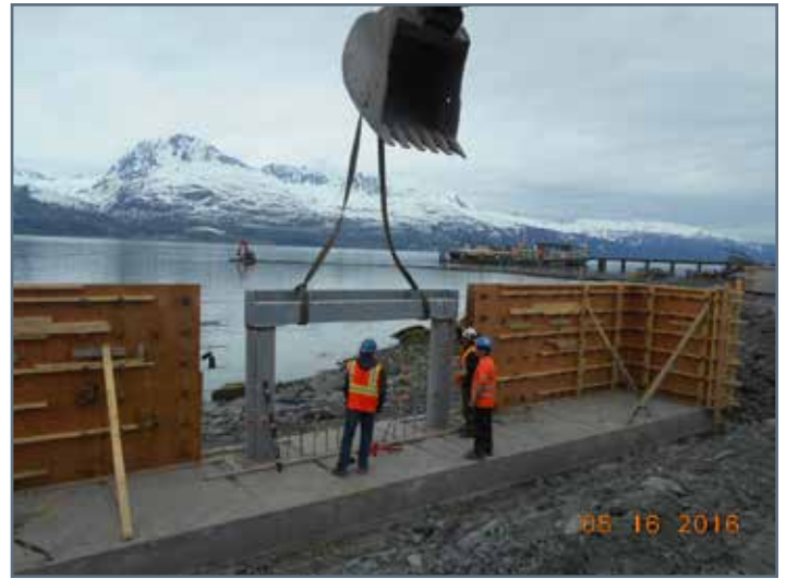
Placing steel cap on piling for attachment of future gangway
