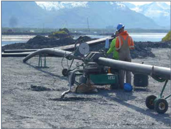
Fusion welding HDPE pipe joints
