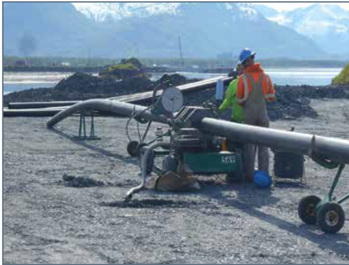
Fusion welding HDPE pipe joints
