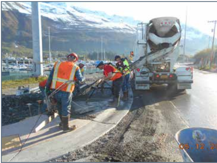
Placing concrete for 8" thick sidewalk area on S. Harbor Drive
