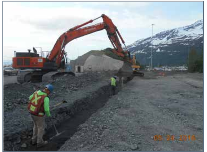
Placing bedding in common trench for electric and telecom
