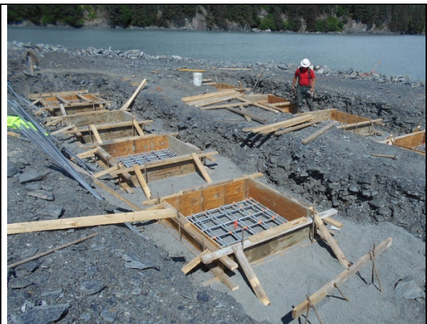
Reinforcement for canopy foundations at East picnic area
