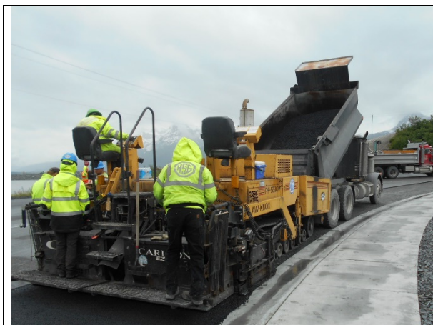
Laying asphalt for drainage transition along new curb & gutter and patch excavation at tie-ins to sewer/water mains
