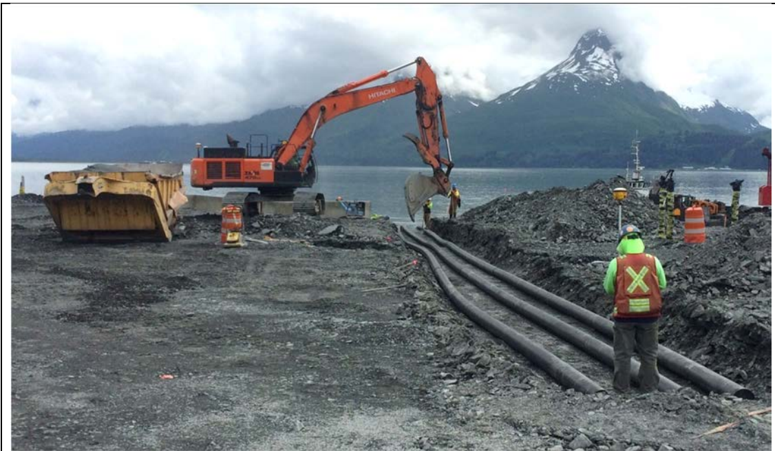
Placing pipes for future contractor/vendor to install fuel and bilgewater lines
