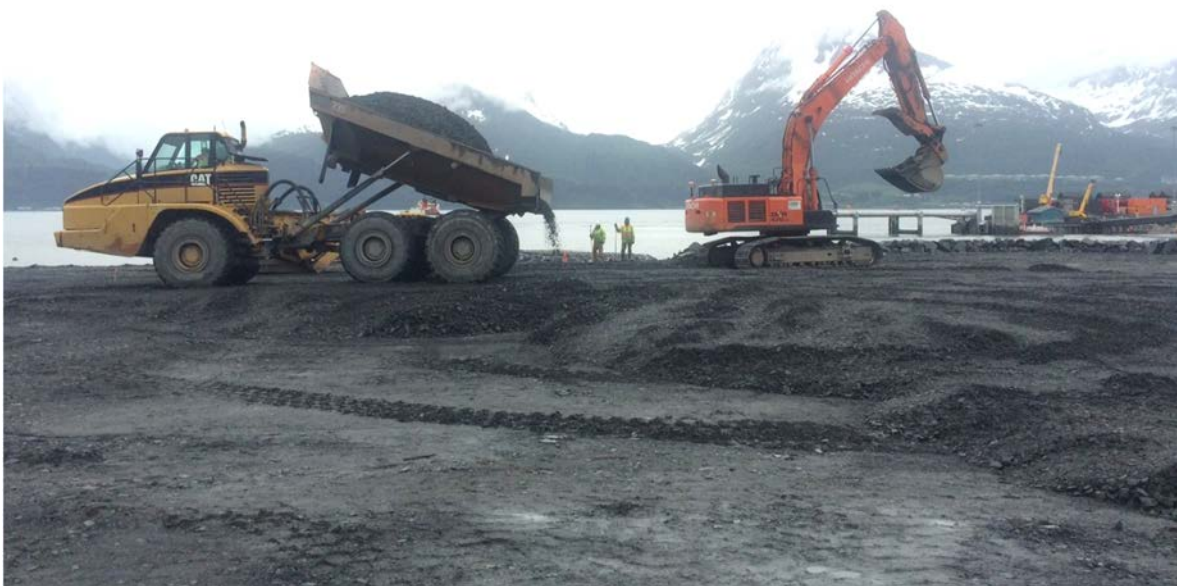
Classified material crushed at Sea Otter is delivered to the site by articulated truck for filling to final grade
