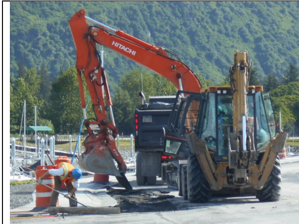
Removing asphalt to provide drainage to new curb & gutter
