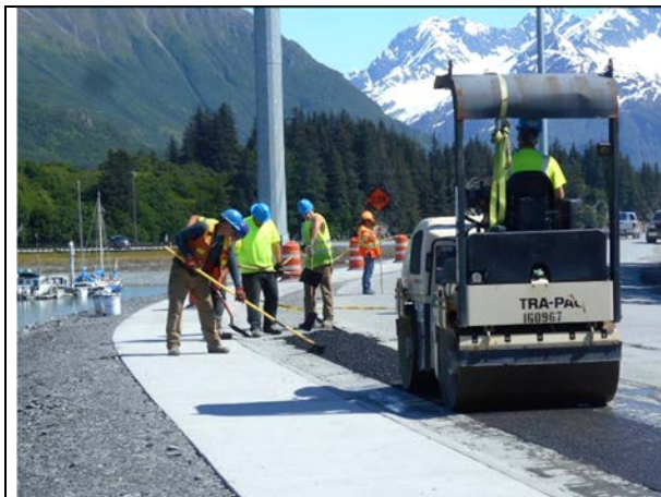
Paving transition from new curb to existing S Harbor Drive
