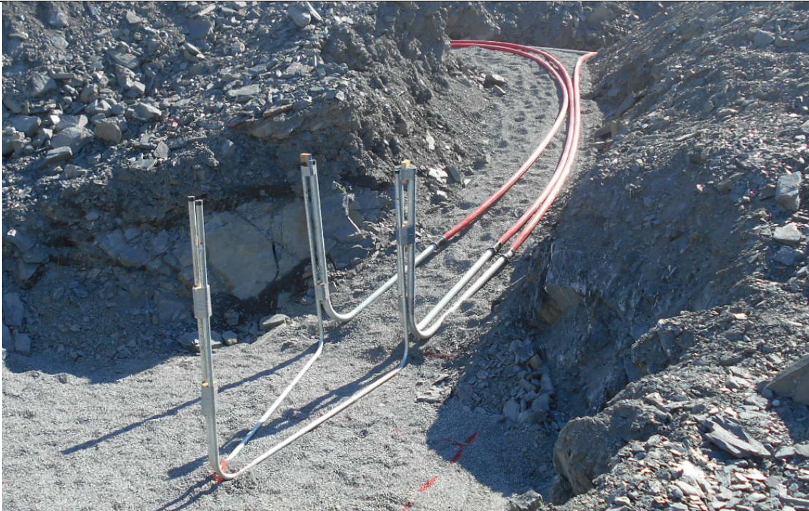
Rigid risers and flexible electrical conduit installed on bedding material in common trench
