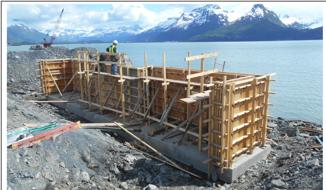
Building scaffolding for placing concrete in retaining wall at Ramp 1 abutment
