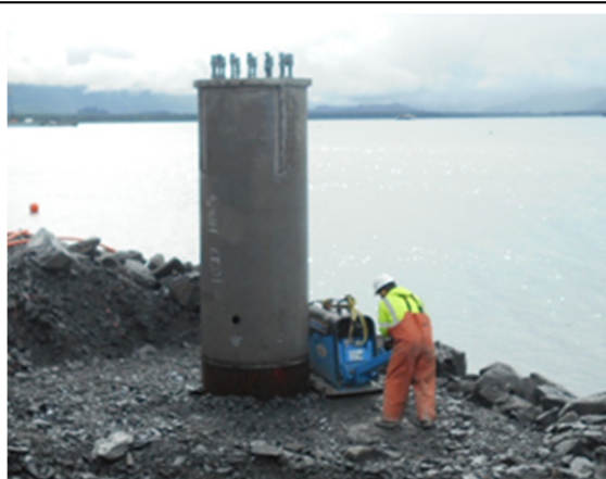
Compacting backfill at high mast light foundation
