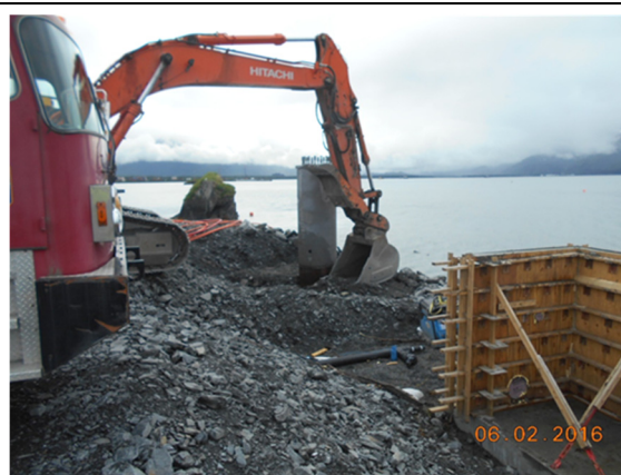
Backfilling around high mast light pole foundation
