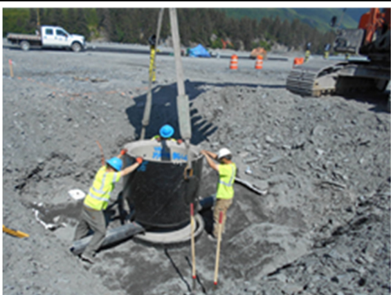
Placing horseshoe section on base for sewer manhole
