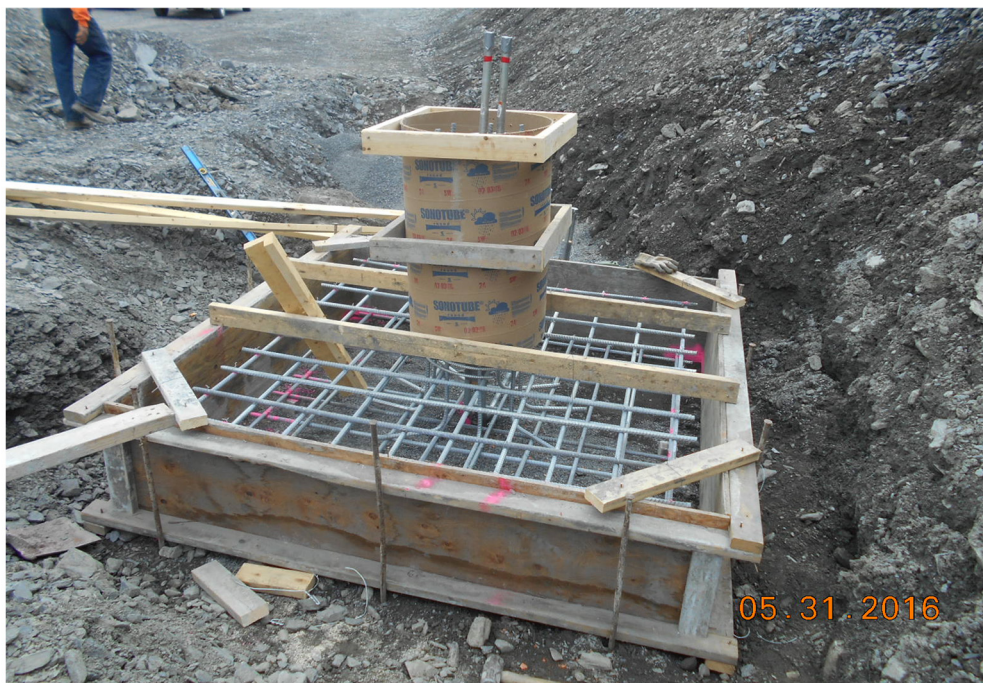
Placing forms and rebar for street light pole foundation
