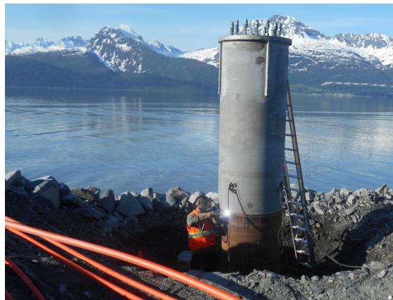
Welding base plate assembly on high mast foundation
