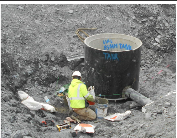
Grouting horseshoe section on sewer manhole base
