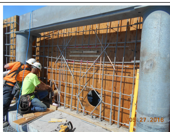
Installing utility penetration thru retaining wall rebar
