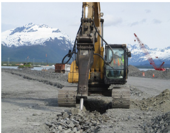
Hydraulic hammer breaking bedrock at utility trench
