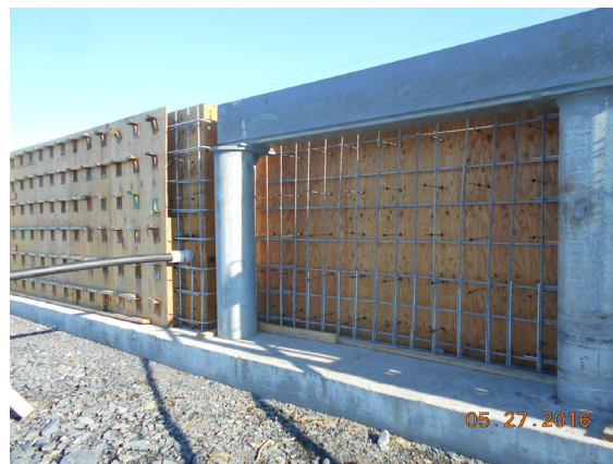
Partially formed retaining wall for ramp abutment
