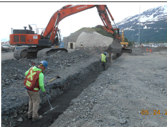
Leveling bedding before laying conduit in utility trench
