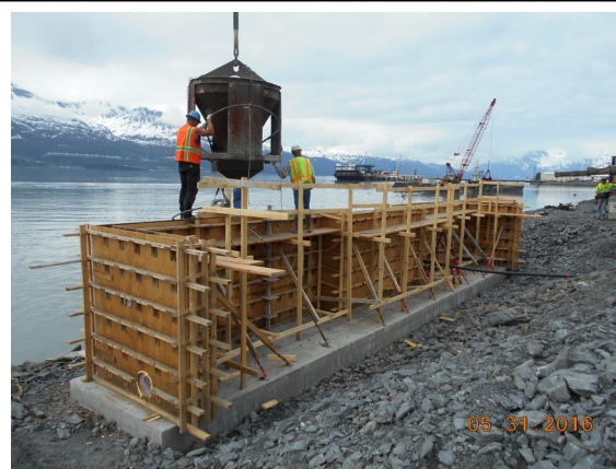
Placing concrete for retaining wall at ramp abutment
