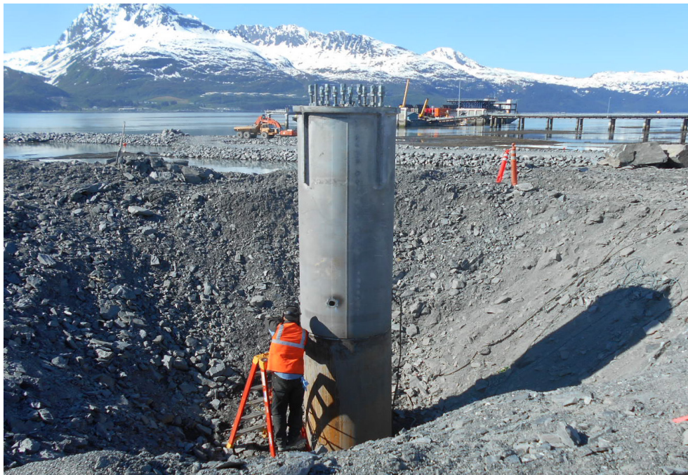
Welding prefabricated hot-dipped galvanized base and pipe section on high mast light foundation pile
