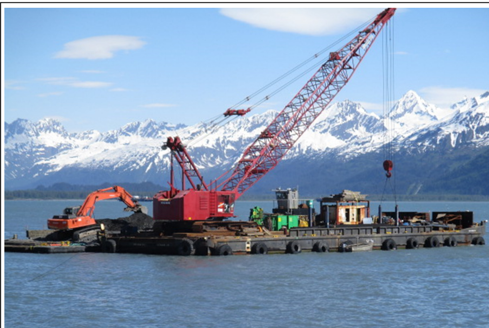
Western Marine barges placing geotextile fabric and filter rock for the east breakwater
