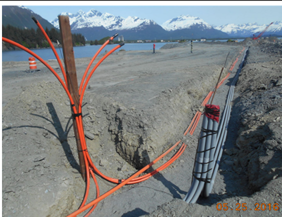
CVEA, CVTV and GCI conduit in common trench
