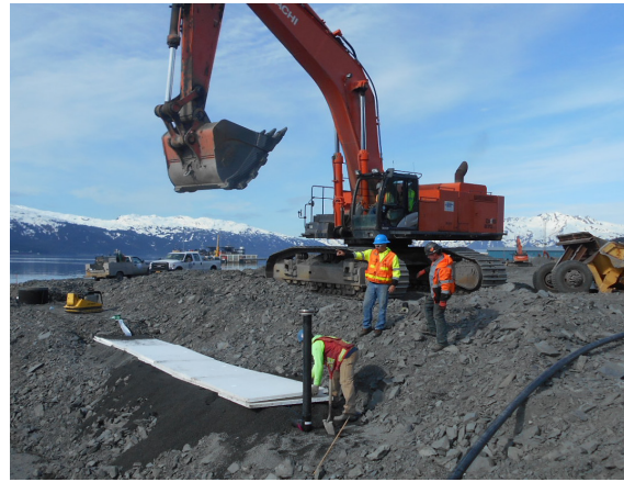
Placing rigid insulation above sewer service line
