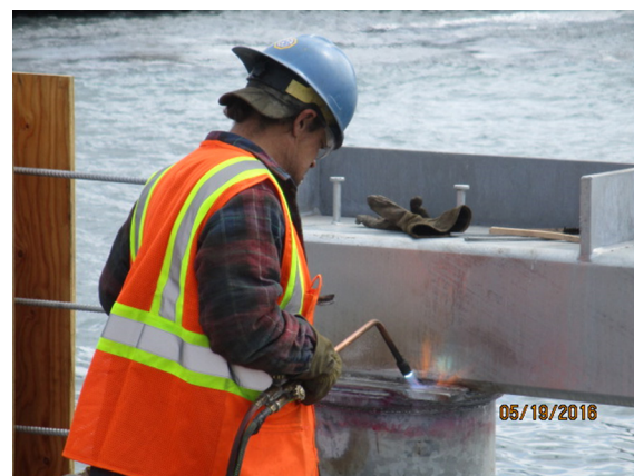
Welding cap on piling for attachment of future gangway
