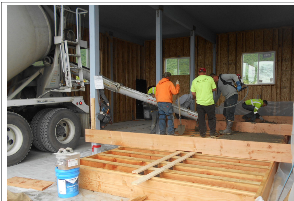
Placing concrete into forms for precast sleepers at Zastrow Enterprises warehouse
