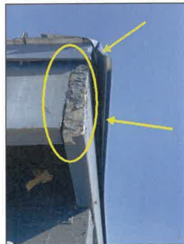
Drip edge is bent out. Fascia is weathered.
