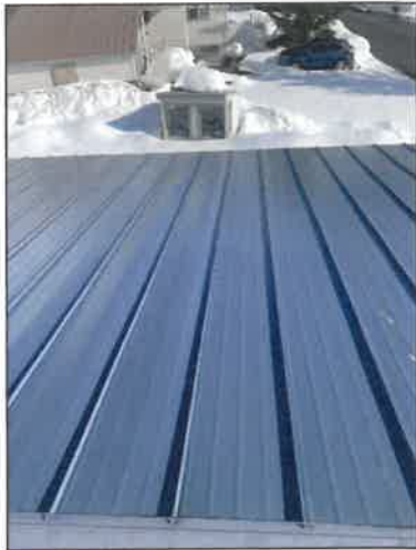
Missing screw on ridge.
