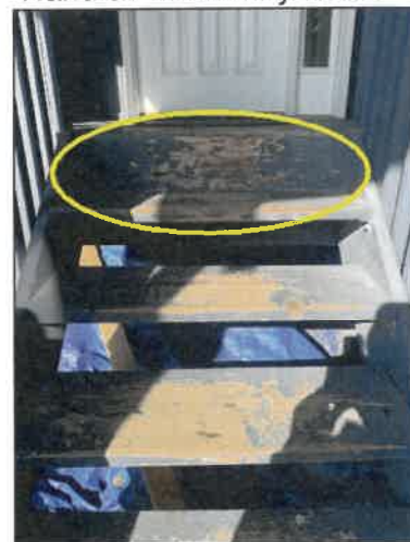
Stairs are not fastened properly to the porch.
