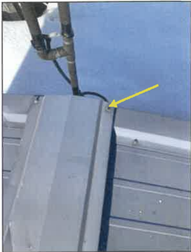
Missing screw on ridge.
