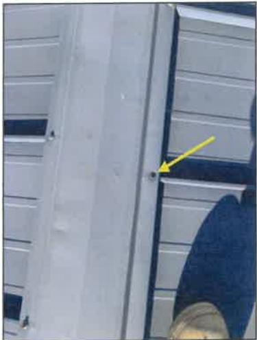
Missing screw on ridge.
