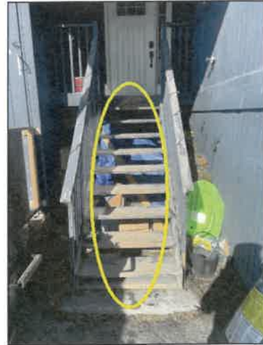
Stairs are worn and weathered. Some steps are damaged.
