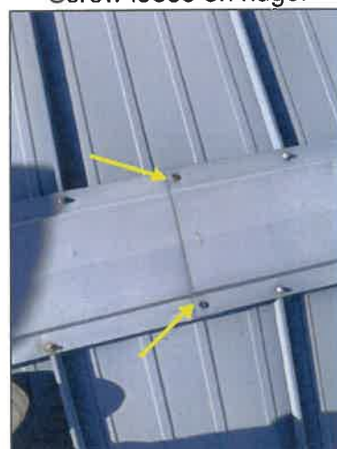
No fasteners on joining of ridge pieces.
