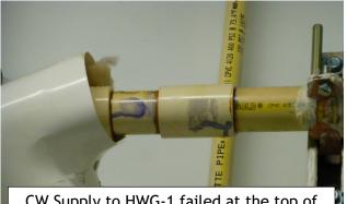
CW Supply to HWG-1 failed at the top of the feed pipe going to the HWG.
