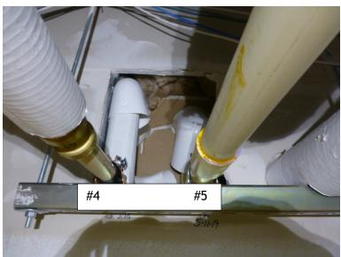
way there was no room for thermal expansion. The pipes continue to run to the south to a space above the boy's locker room. Plans 1/M222 and 2/M222 show a 28" offset
