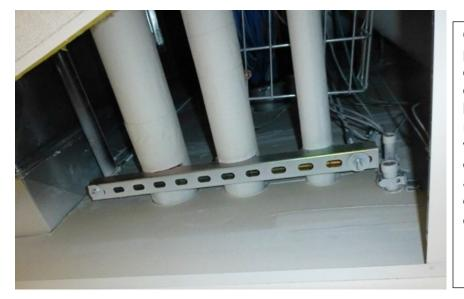
CW, HW, HWC piping above drop ceiling in corridor outside entry to boys' locker room. Piping with offset expansion loop is above hard ceiling and is concealed.
