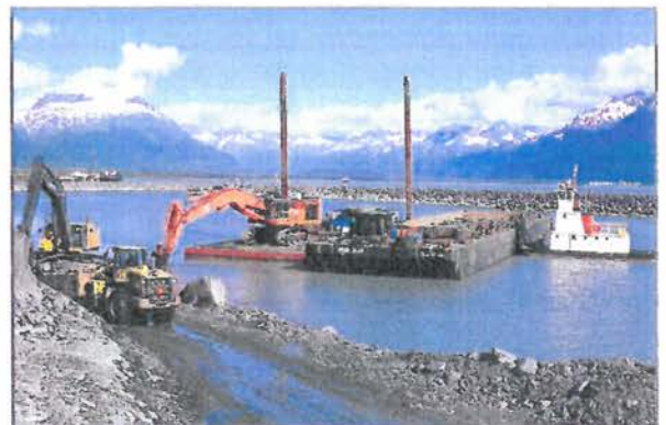
Tug Halle helps position barges while EX1200 dredges shot rock and places in bottom dump barge
