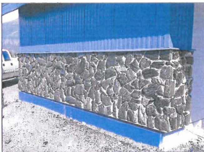
Rock around East Restroom was pressure washed and sealed
