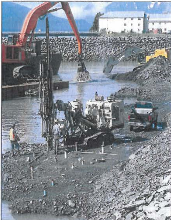
Drilling holes for blasting rock at west end of mooring basin while excavators dig material and load on the dump barge
