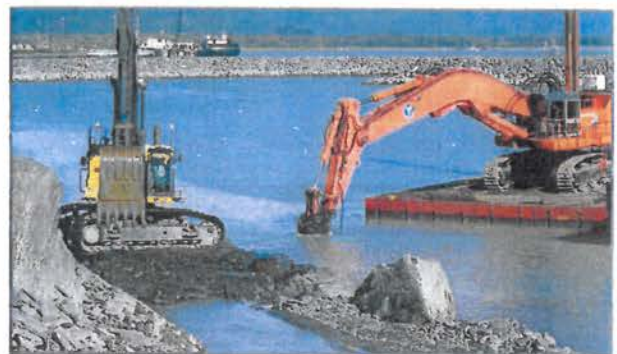
EX1200 on barge uses hydraulic hammer to break bedrock below water
