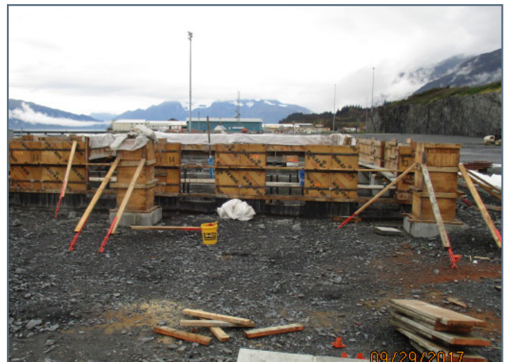
Warehouse Building – Concrete placed in stem wall and pier forms
