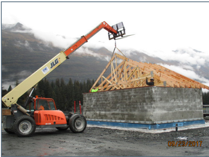
East Restroom – Setting roof trusses
