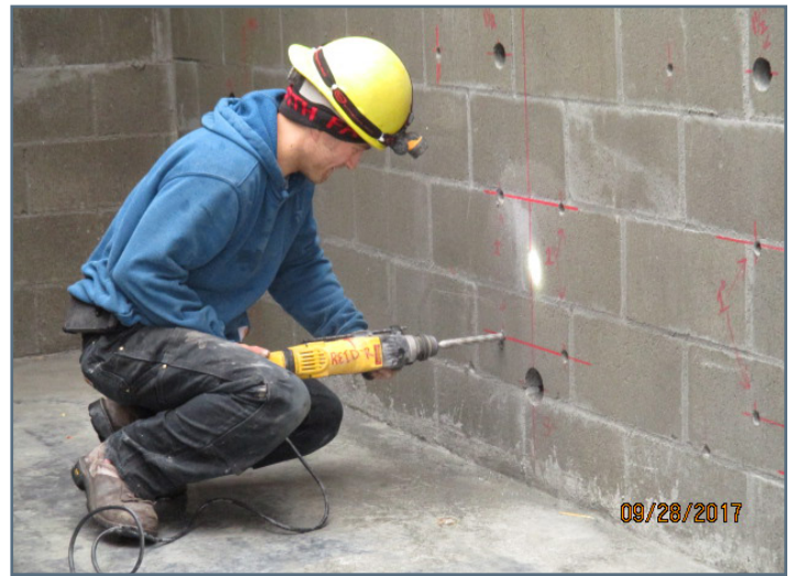
Restroom - Drilling holes for securing concrete core drill
