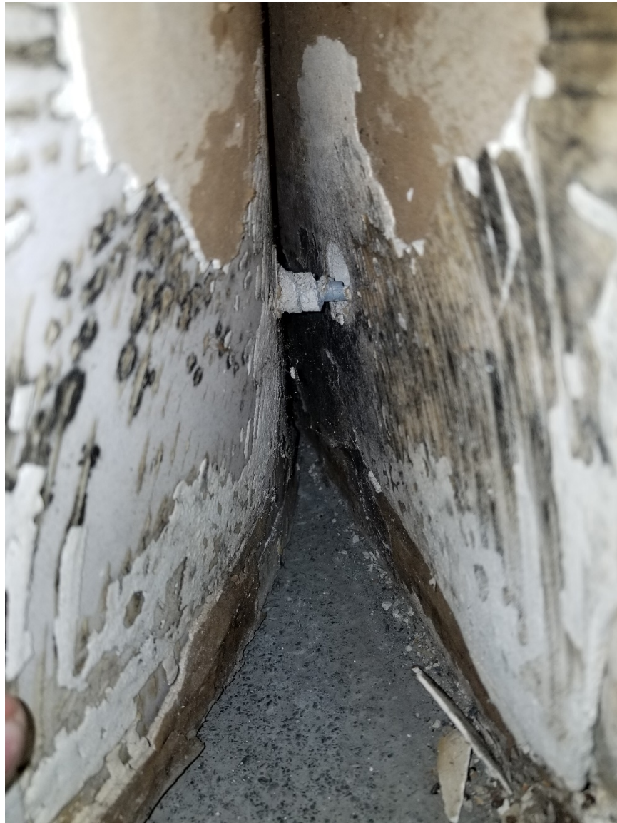
Mold growth on wall system and base of wainscot
