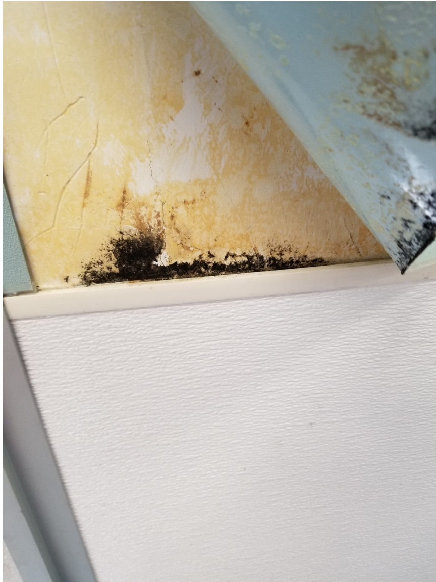
Mold growth on wall system and Mylar wainscot located at the top seam, typical design throughout the kennel
