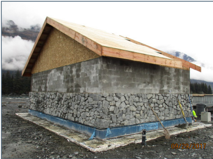
Restroom - Walls, stone veneer installed; roof partially sheathed
