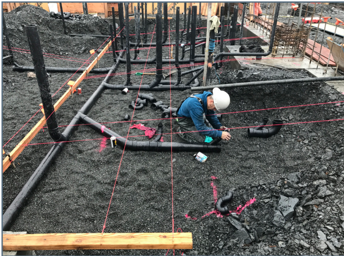
Warehouse Building - assembling waste piping below floor grade
