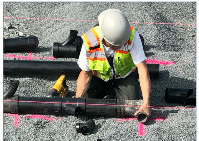
Bilge Treatment Building - assembling waste drain pipe below slab
