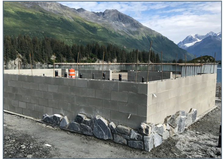
Restroom - Temporary rock veneer mock-up for City review
