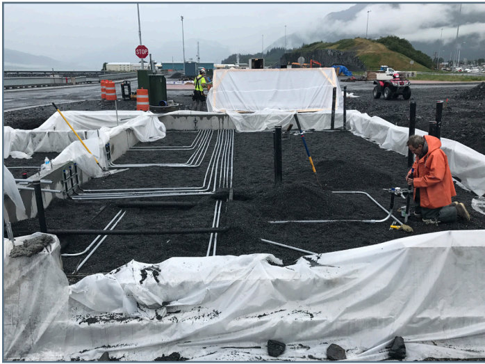
Bilge Treatment Building - installing electrical conduit below floor
