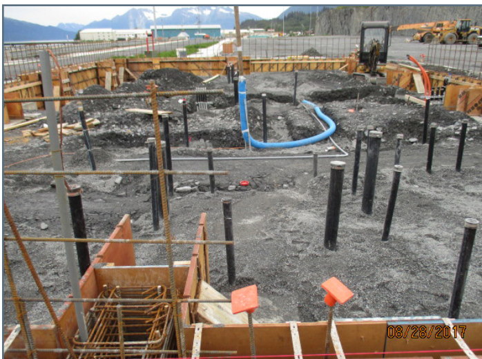
Warehouse Building - plumbing/electrical roughed-in, stubbed up for floor slab
