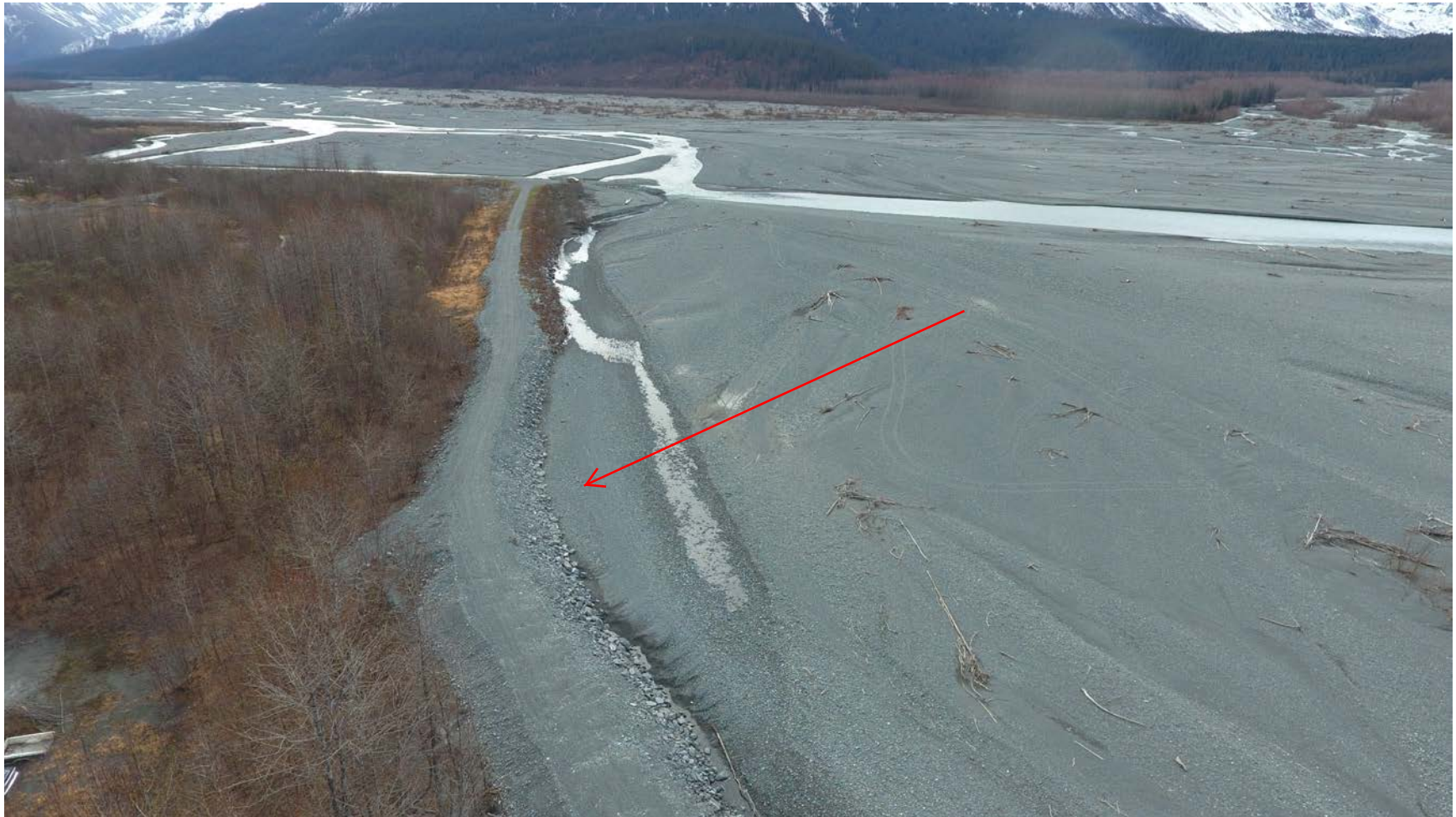
An oblique view of groin #4 looking upstream at the area to receive riprap.
