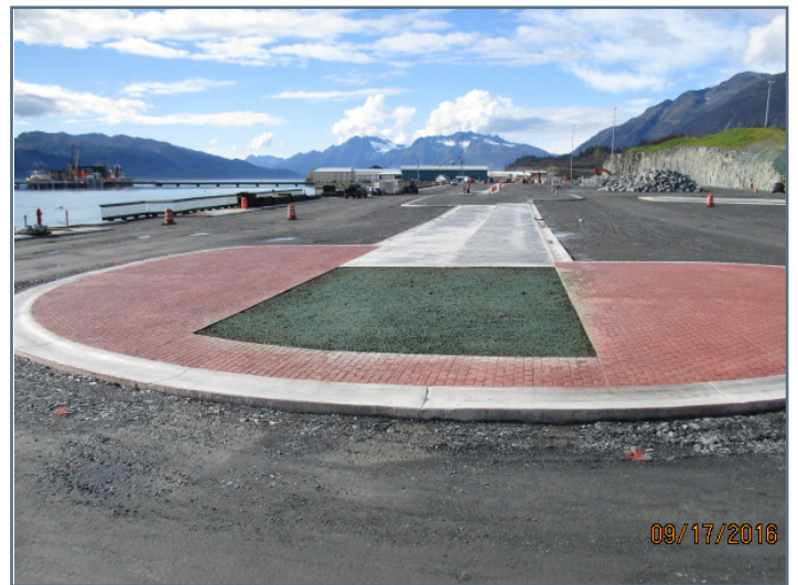
Brick imprinted concrete and topsoil separate access road traffic from parking spaces at east end of site
