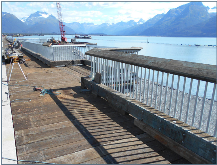
Installing timber top rail on steel guard rail assembly
