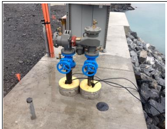
Installed backflow preventer (BFP) at Ramp #3
