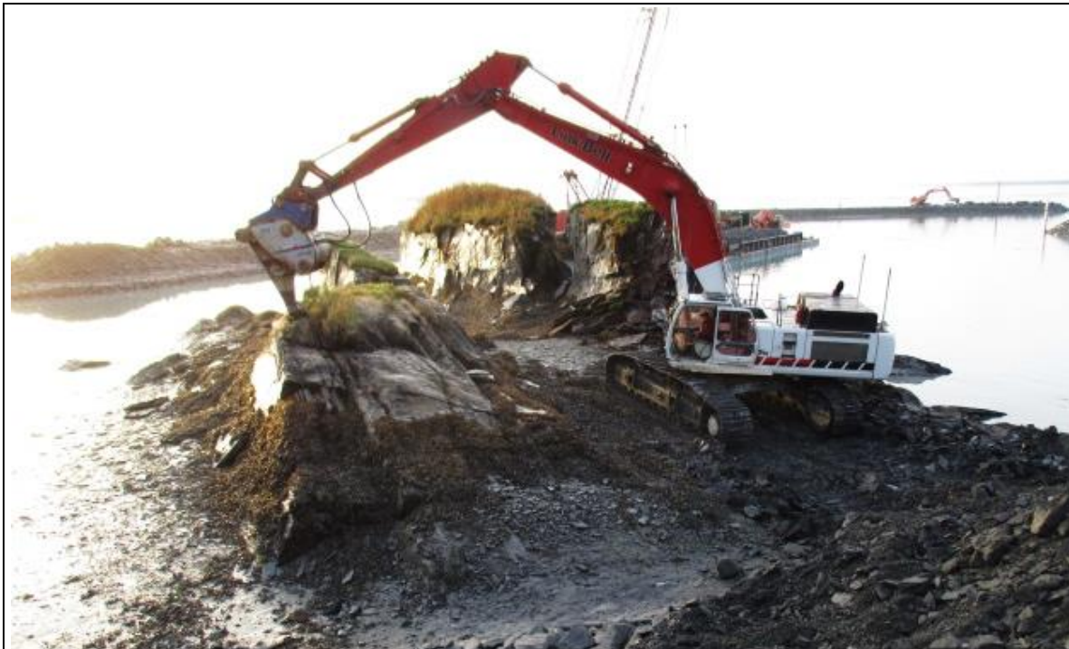
Testing Xcentric Ripper ability to break bedrock at rock outcrops in proposed Drive-Down Float basin
