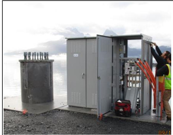
Installing electrical cabinets near east ramp (#3)
