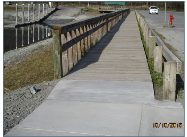
New transition from existing boardwalk to sidewalk
