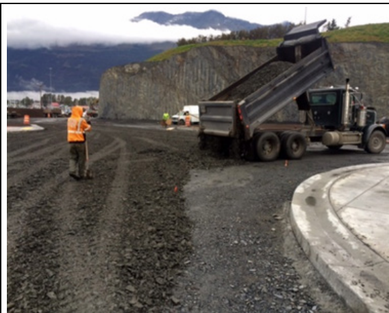
Delivering Type II-A gravel for final subgrade
