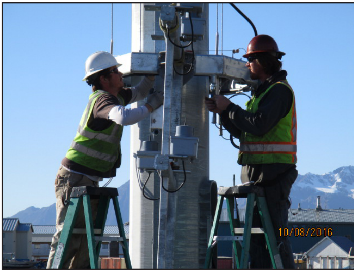
Installing high mast light fixture array
