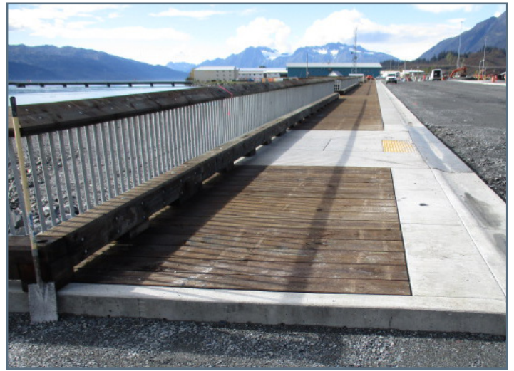
Typical boardwalk view with handrail and curb
