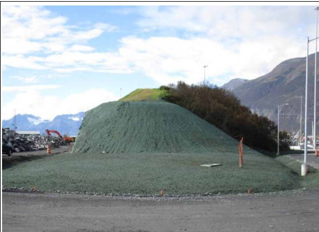
Topsoil hydroseeded at East end of Hotel Hill; street lights installed along East Access
