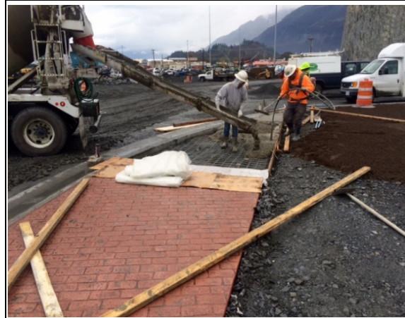
Placing standard sidewalk next to brick imprint
