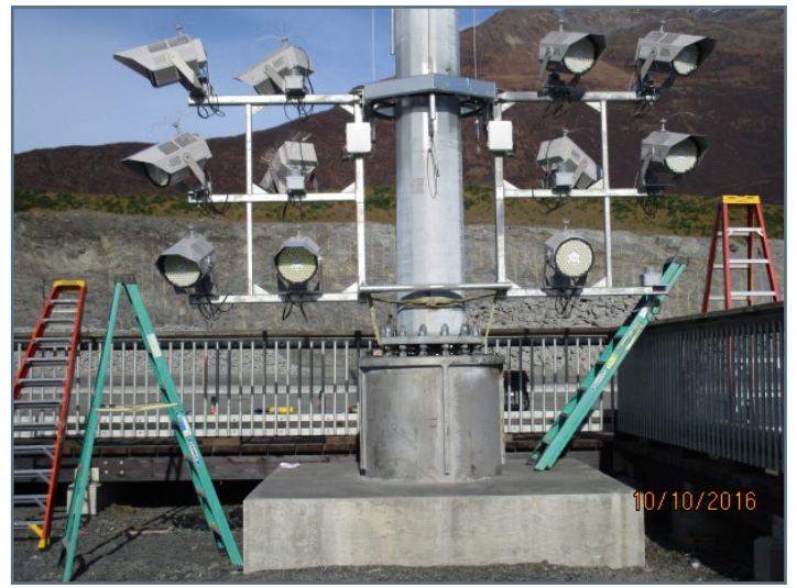
High mast light arrays with LED light fixtures
