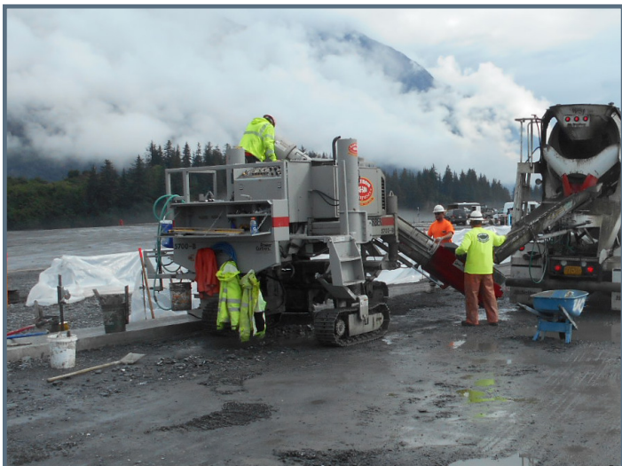
Slipform machine placing concrete for curb and gutter
