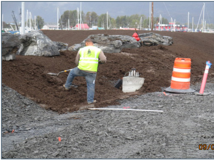
Spreading topsoil on berm at west property line
