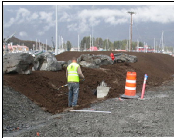
Spreading topsoil on berm along West Access
