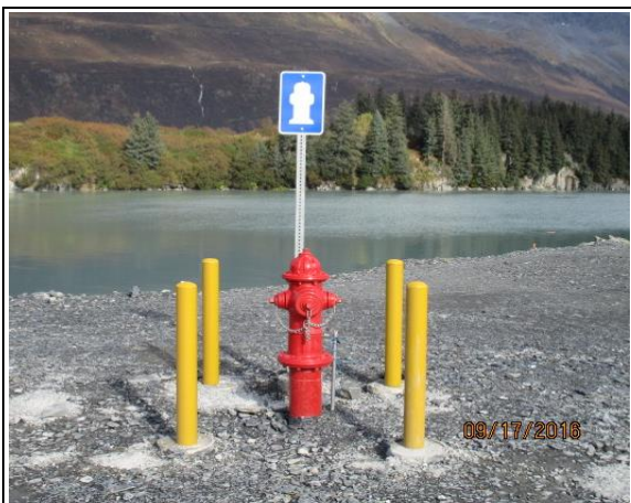
Protective bollards and sign installed at hydrant
