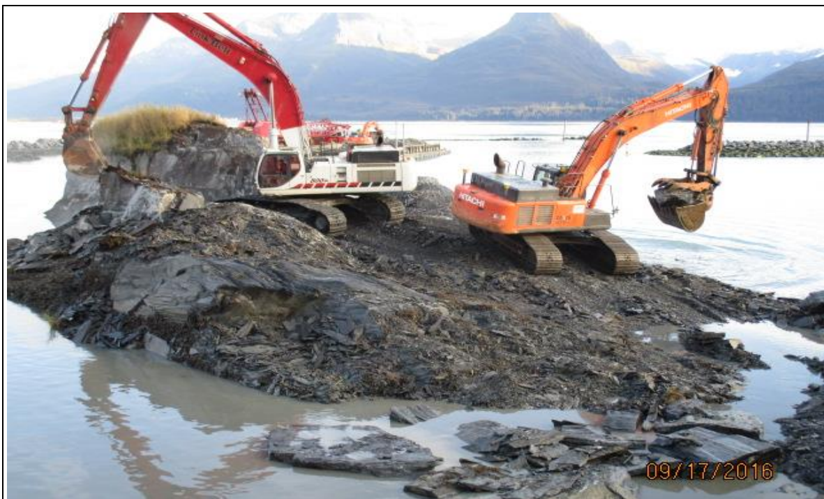
Hoe with rock bucket (left) breaks bedrock while hoe with “thumb” places large rocks for future drill pad
