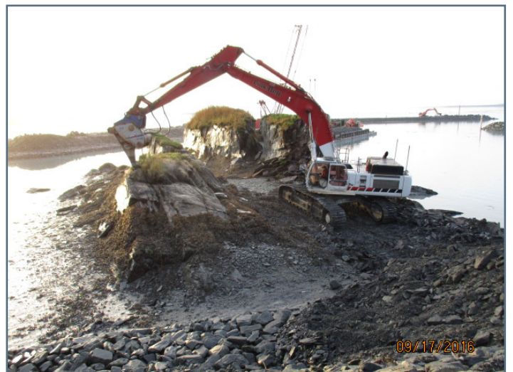
Xcentric ripper test on rock at east end of fill
