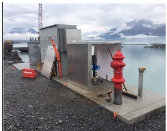
Assembling insulated/heated enclosure around BFP
