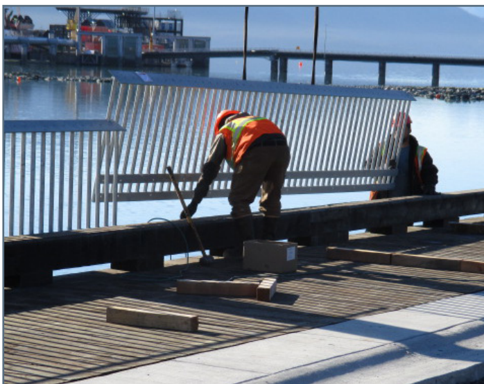
Placing guardrail for the boardwalk
