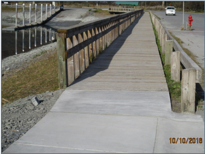
New transition from existing boardwalk to sidewalk
